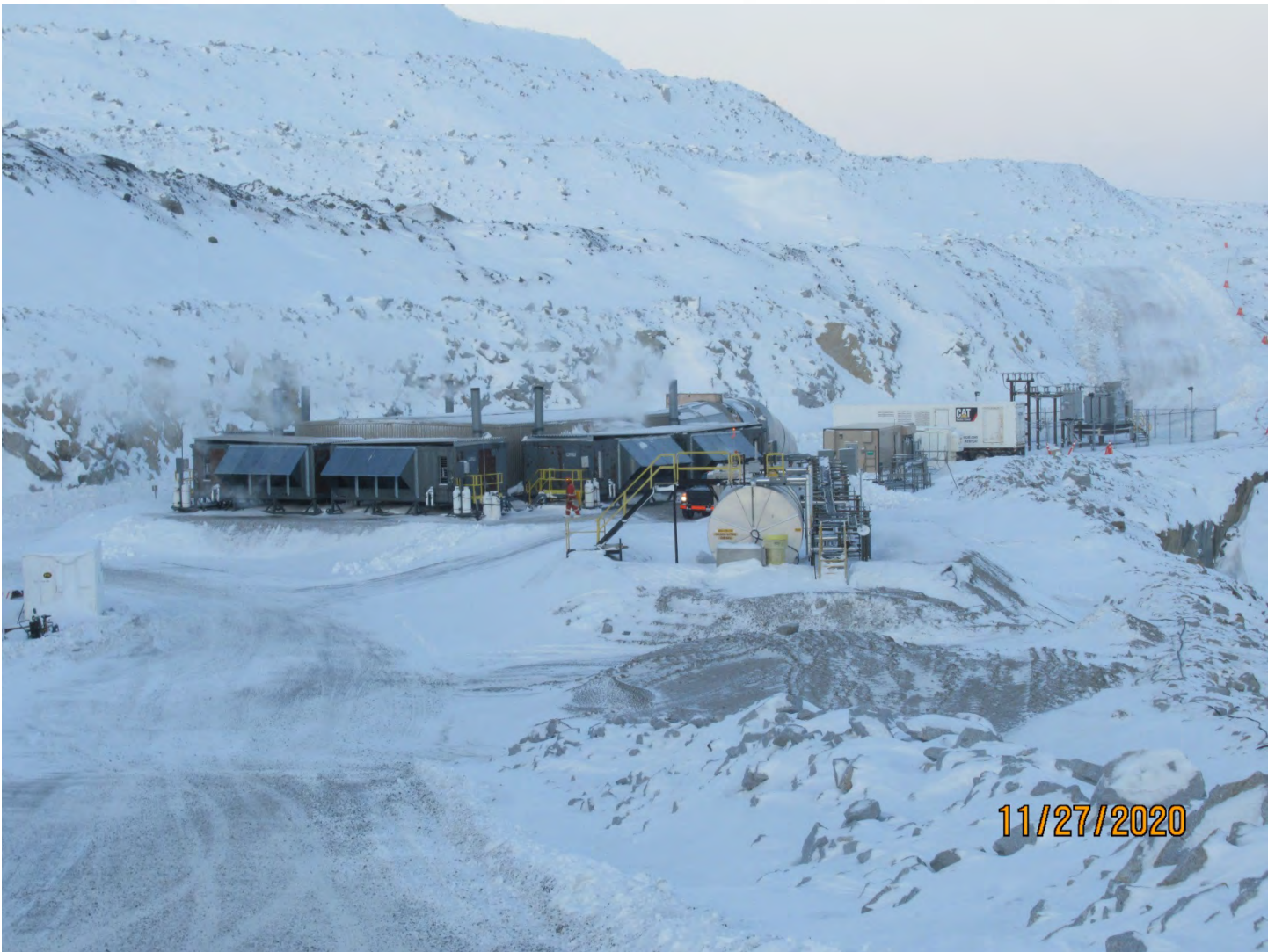
Photo 3: The FAR on the Misery Pit 440 Bench has been commissioned along with the electrical to the underground. A backup generator has also been installed in the event of electrical failures.
