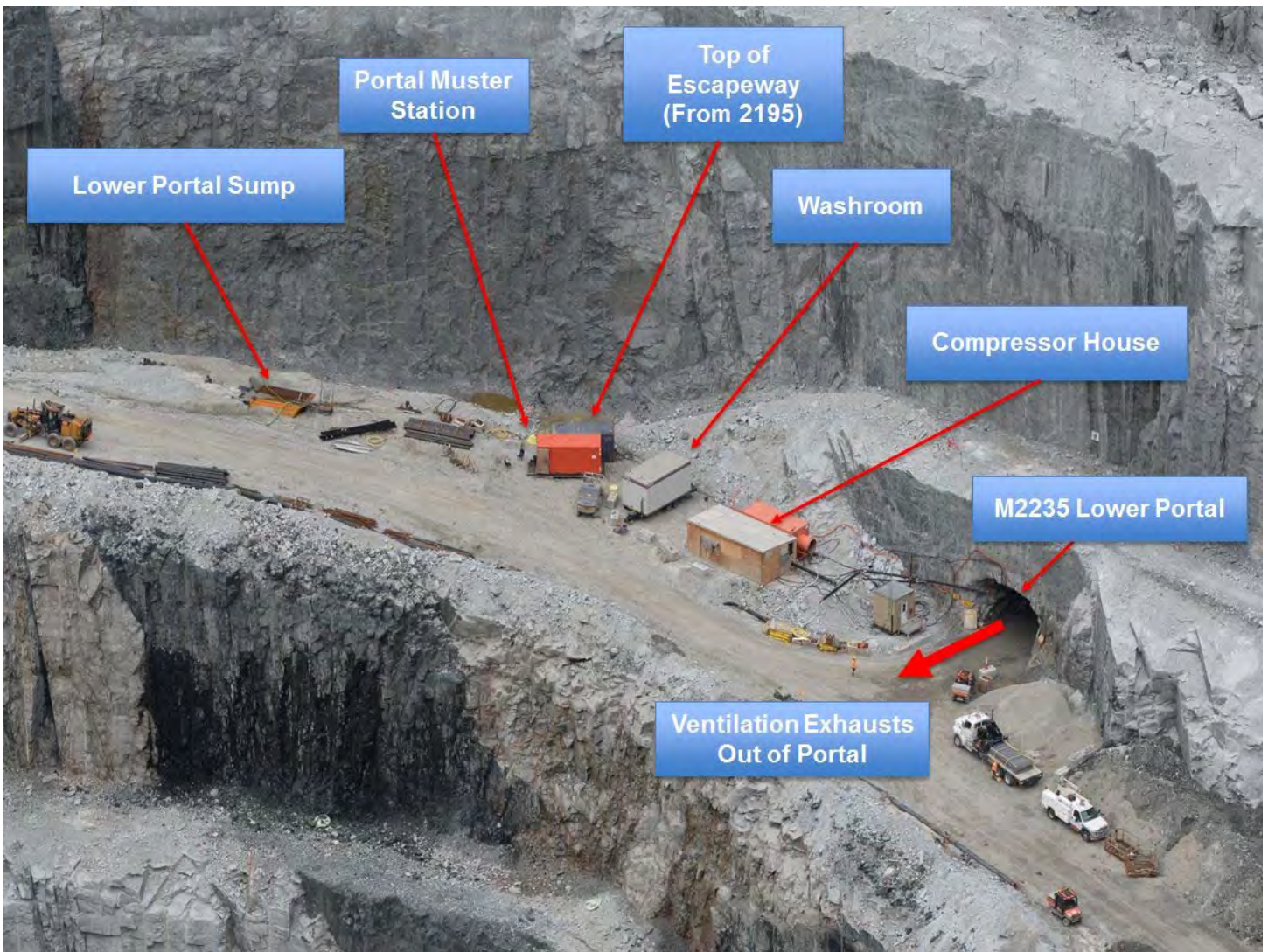
Photo 5: As seen in this photo, the majority of the equipment staged on the 2235 Lower Portal ramp was removed as it was no longer required to support the underground mining activities.
