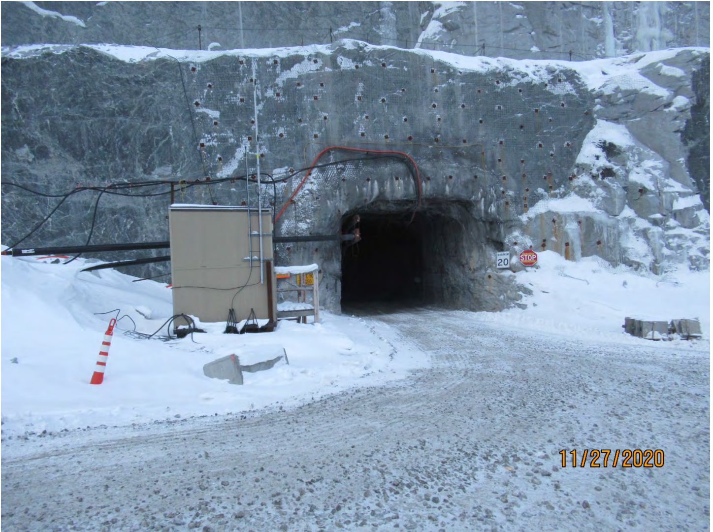
Photo 11: Heated air and vent lines have been removed at the 2235 Lower Portal as they are no longer required.
