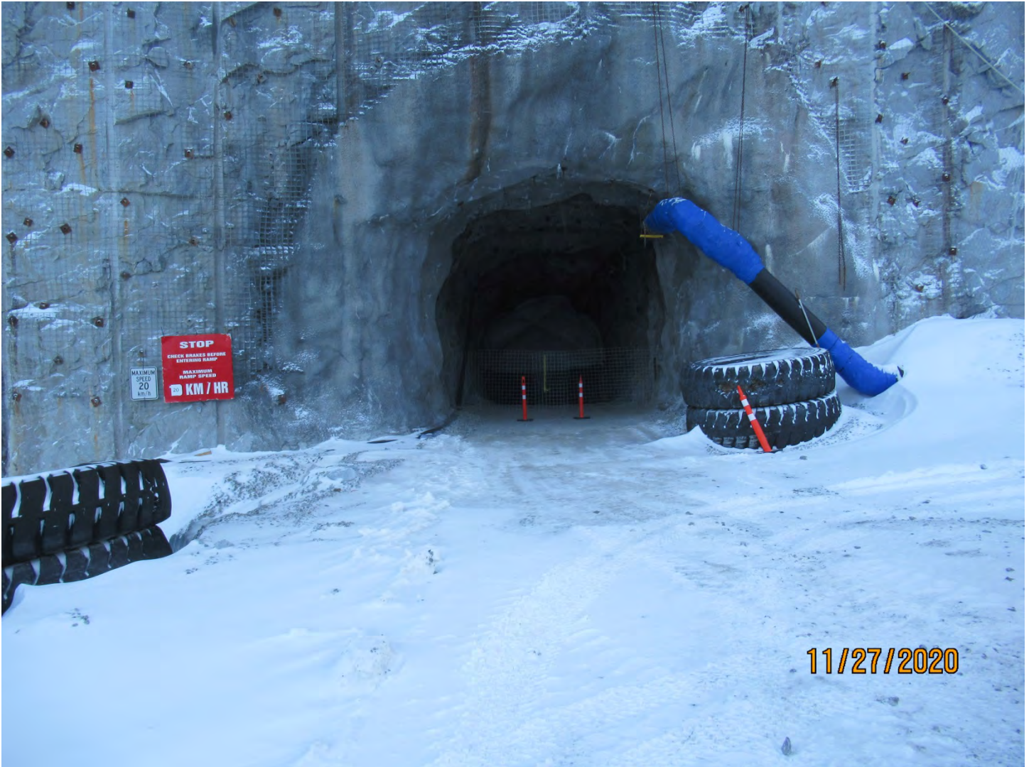
Photo 1: A heat-traced water line is used to discharge water into King Pond via the 2340 Upper Portal.
