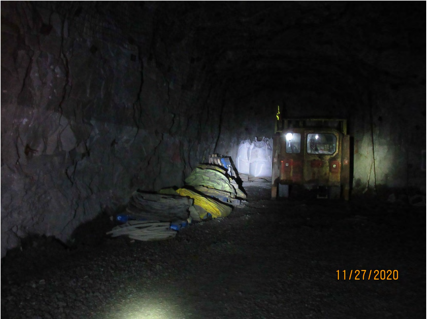
Photo 23: Bags of shotcrete and soft vent lines are also being staged at the U/G 2120 Level.
