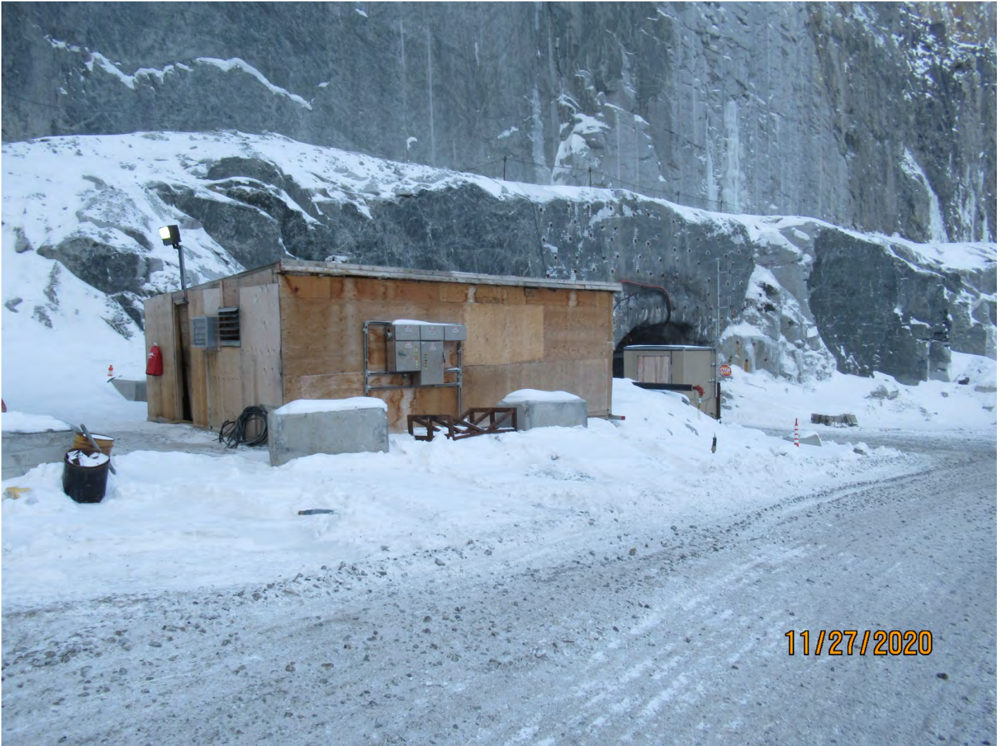
Photo 9: Compressors on the 2235 Lower Portal ramp will remain in use until a compressor station is established at the U/G 2150 Level.
