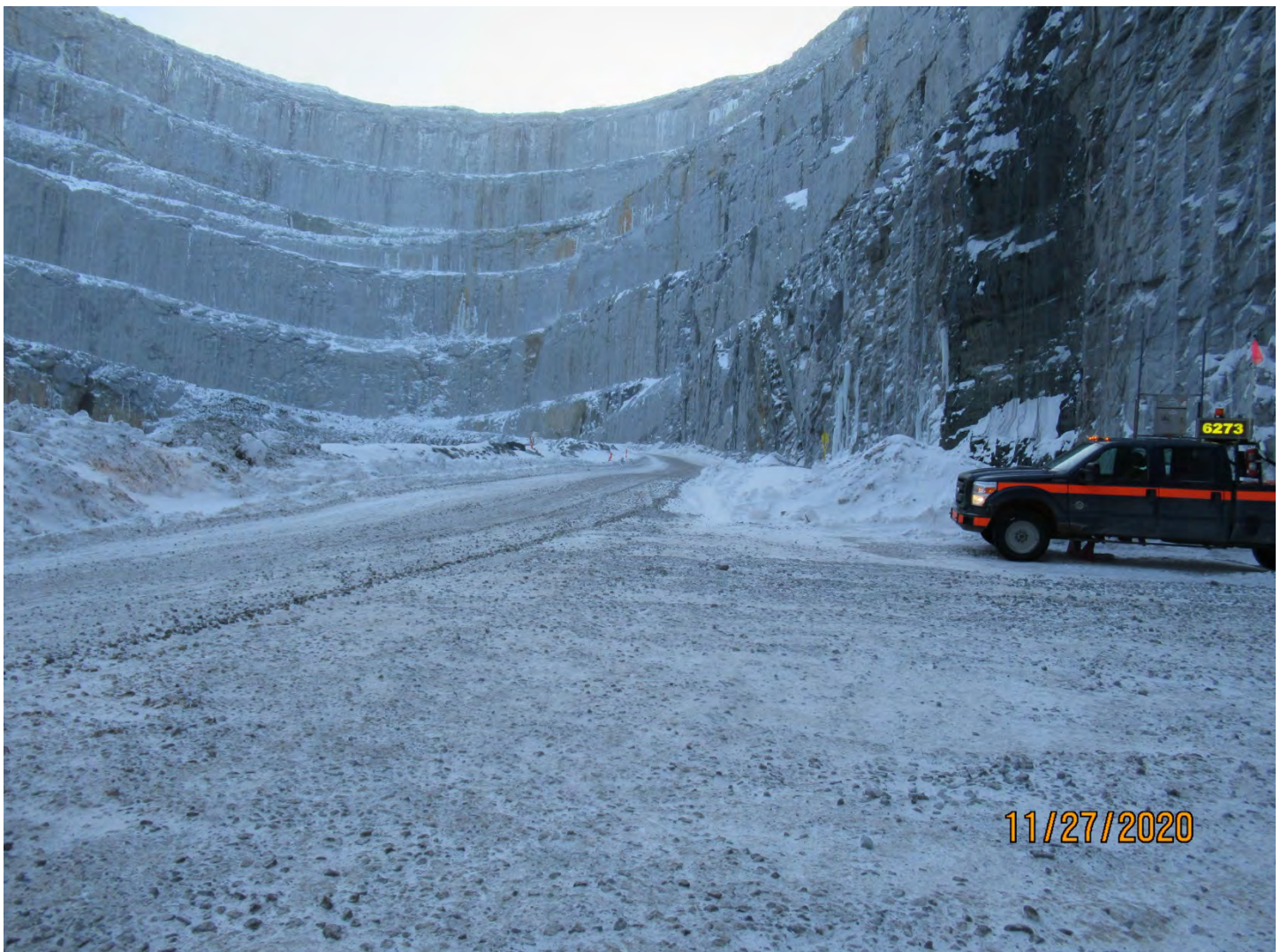
Photo 6: As seen, fuel tanks, generators and other equipment are no longer present on the 2235 Lower Portal ramp.
