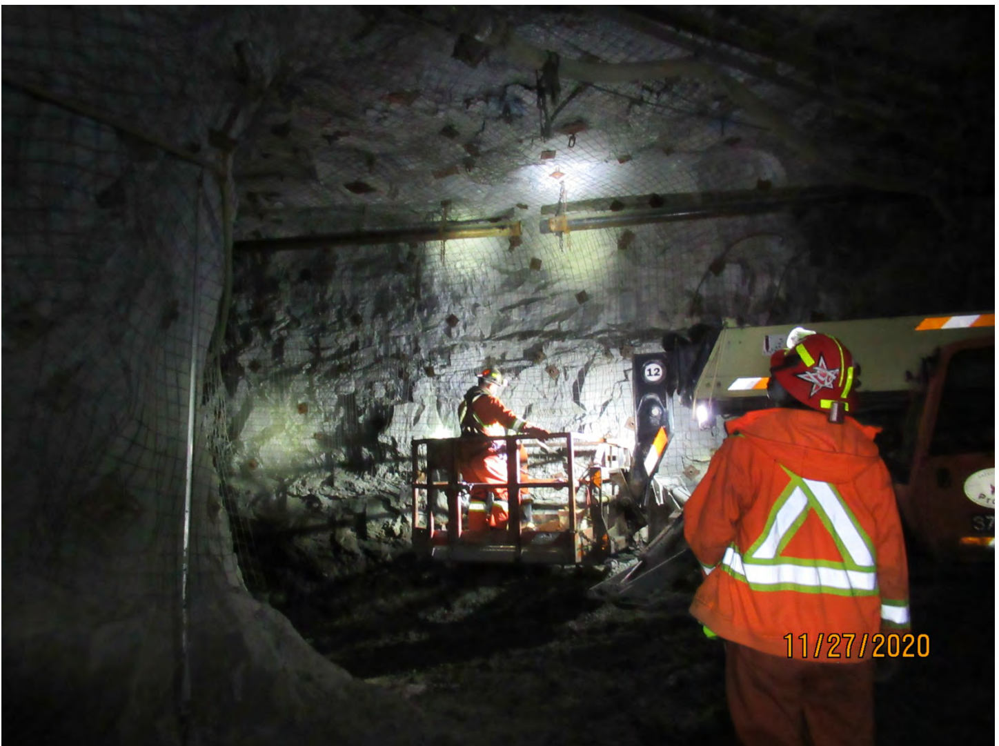
Photo 18: Crews were plumbing in water lines at the U/G 2100 Level.
