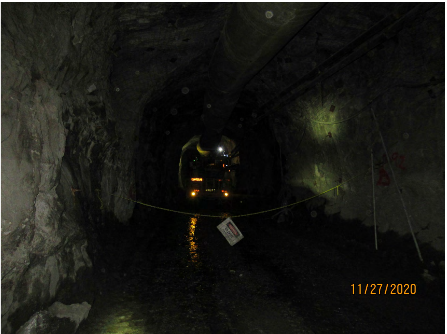
Photo 20: This Maclean Bolter was being used to hang screen at the U/G 2100 Level as part of the ongoing drift rehabilitation work.
