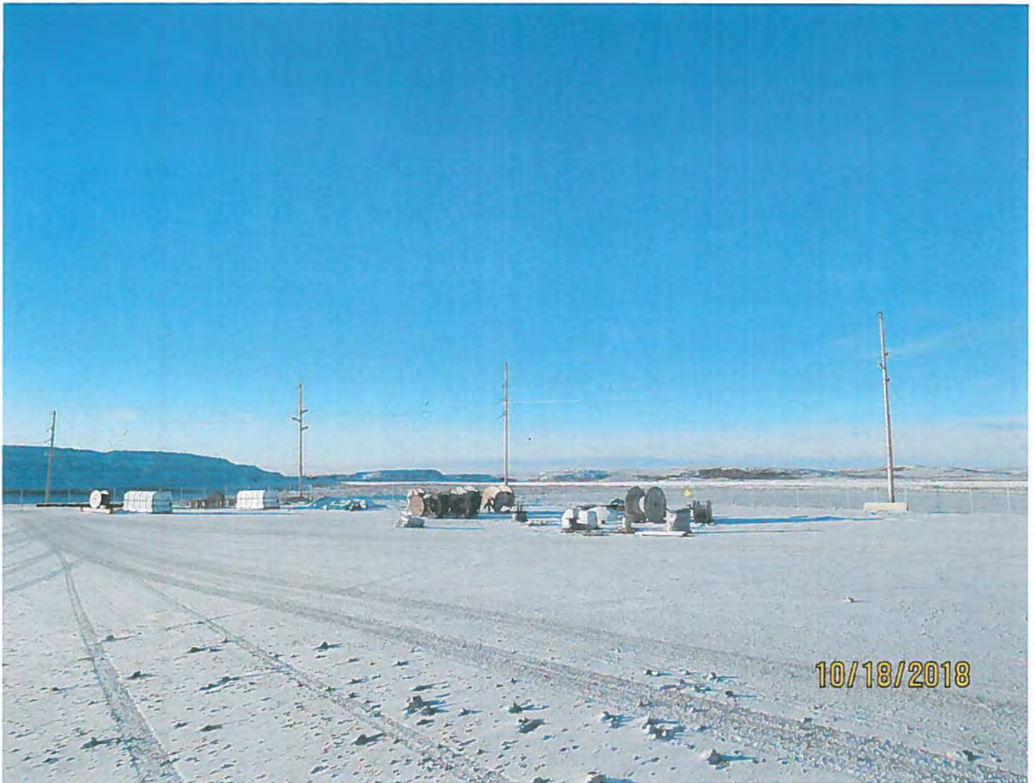
Photo #7 - W2017D0004 MUG Project There were a minimal amount of materials staged in laydown in the northeast of the Misery Camp compound.
