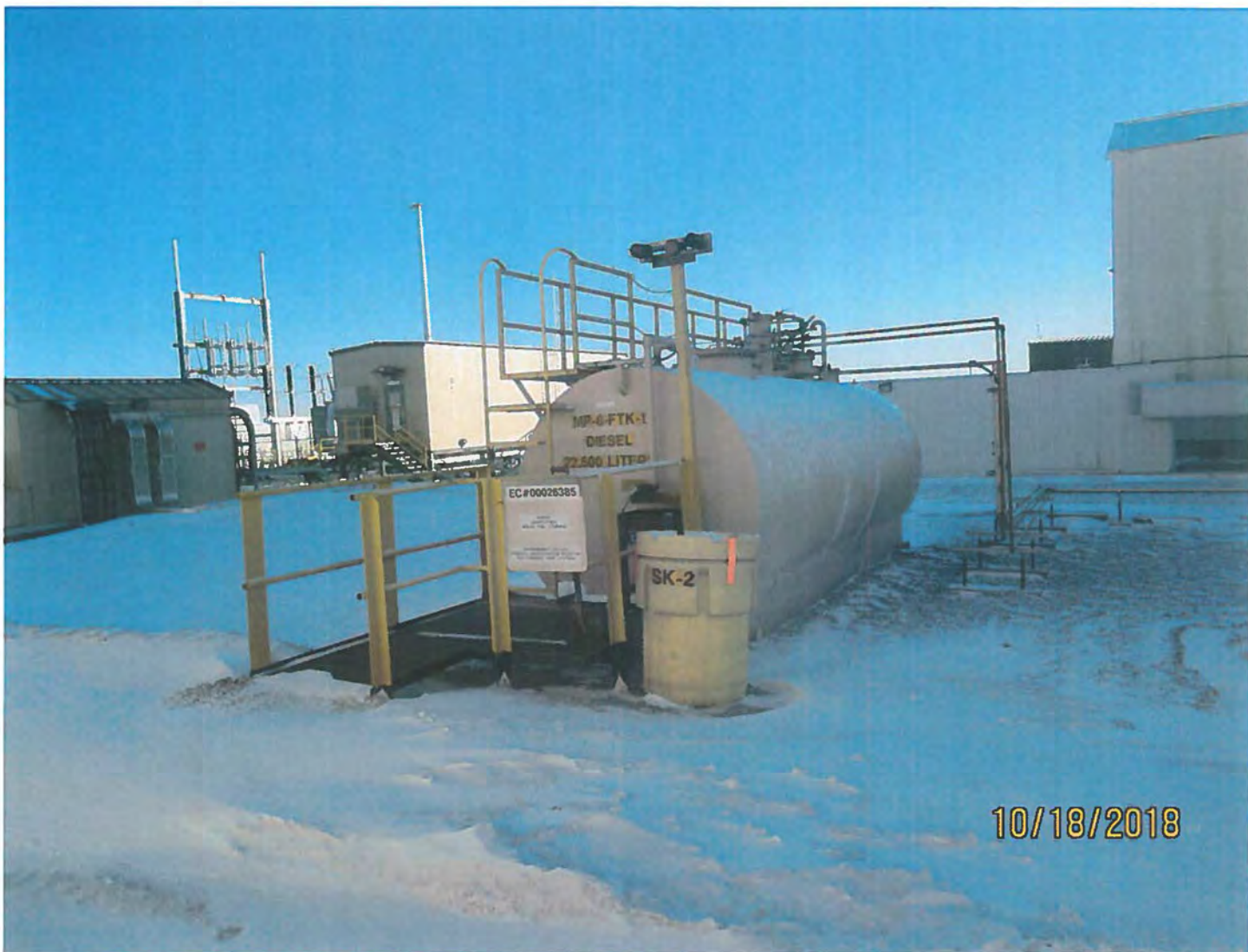
Photo #23 - W2017D0004 MUG Project An example of a fuel tank in containment with readily available spill response materials.
