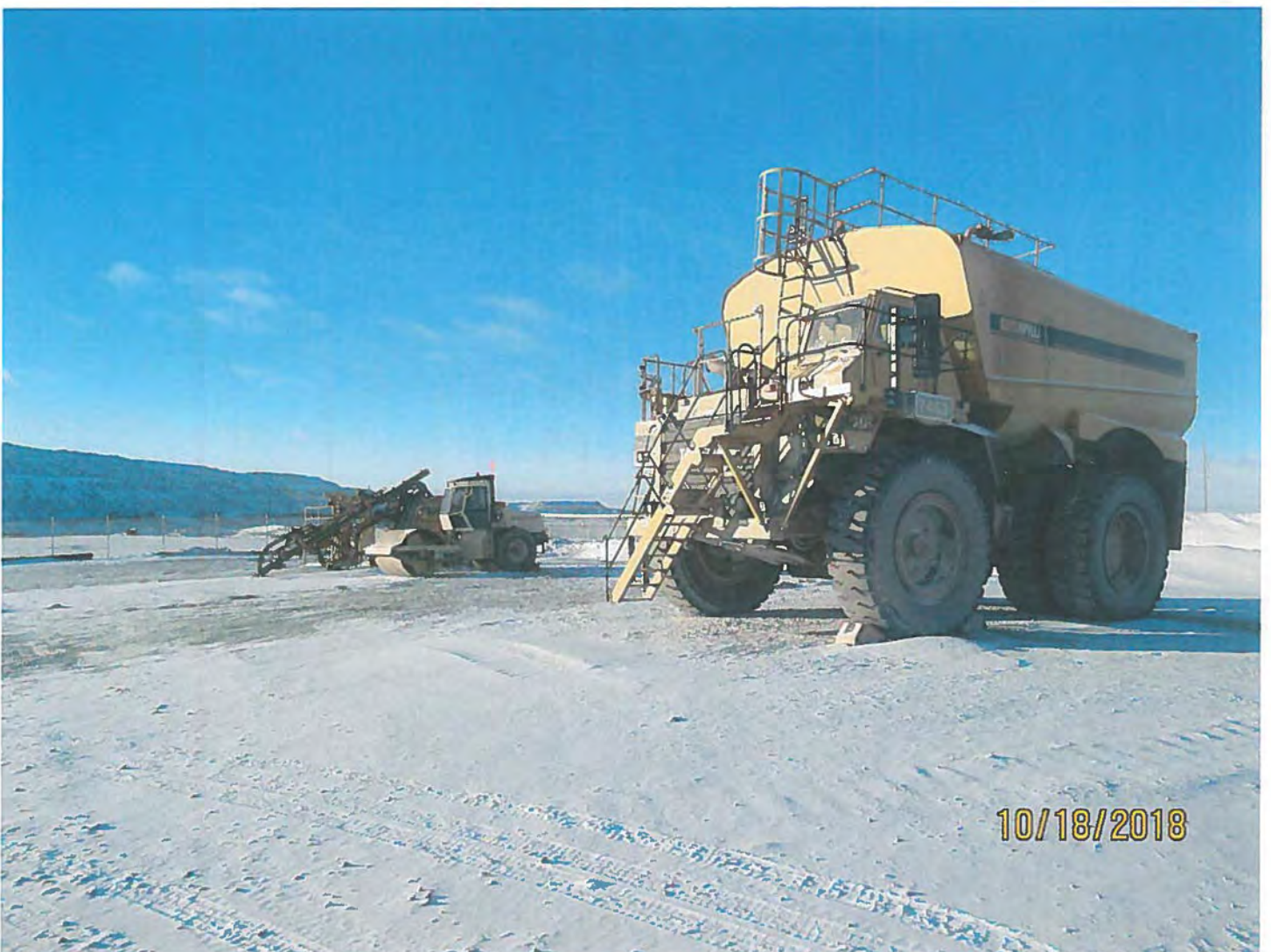
Photo #8 - W2017D0004 MUG Project Looking north at the heavy equipment laydown.
