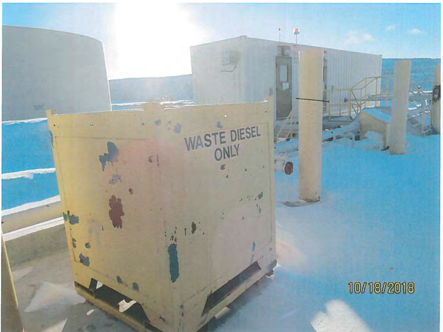
Photo #22 - W2017D0004 MUG Project Waste diesel collected at the fuel offload station is placed in this holding container.
