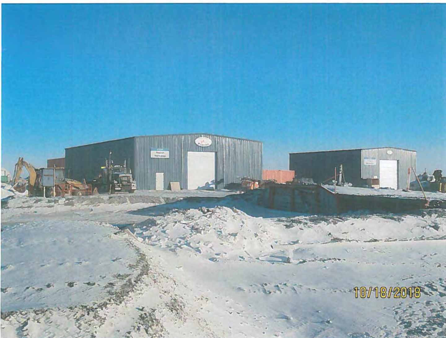
Photo #4 - W2017D0004 MUG Project The welding shop (left) and cold storage building (right) are located on the west of the Misery Camp compound.
