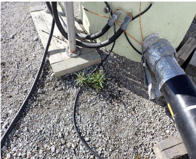
Photo 3: Misery Camp Lift Station – View of cleaned up spill site after enzymes application and evaporation.
