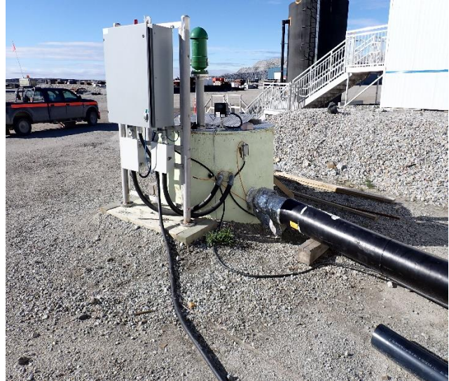
Photo 2: Misery Camp Lift Station – View of cleaned up spill site after enzymes application and evaporation.
