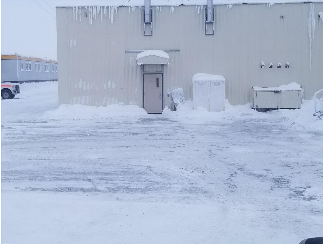
Photo 2: After photos of Spill-2023519 at Misery Camp.
