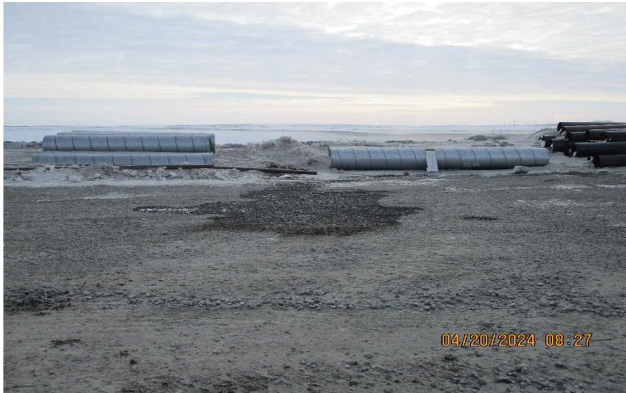
Photo 1: Before photo of Spil-2024114 at Misery Crusher Pad.
