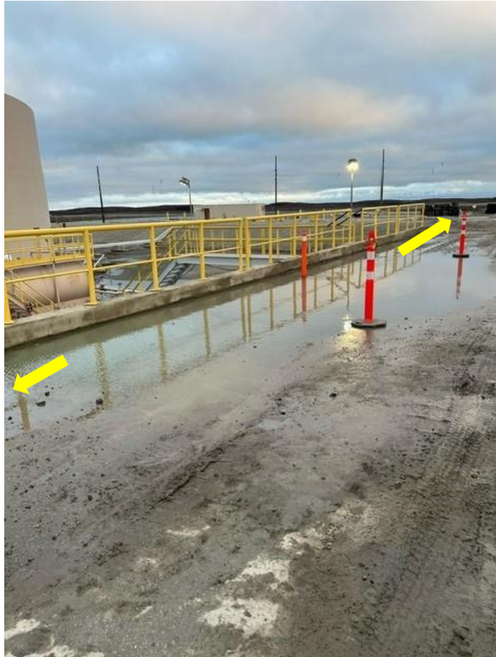
Photo 2. View of the subsurface sump that overflowed due to rainwater mixed with diesel. The arrows highlight the flow of diesel/water from the paved product transfer area onto compacted gravel adjacent to the fuel station. Photo facing northeast.
