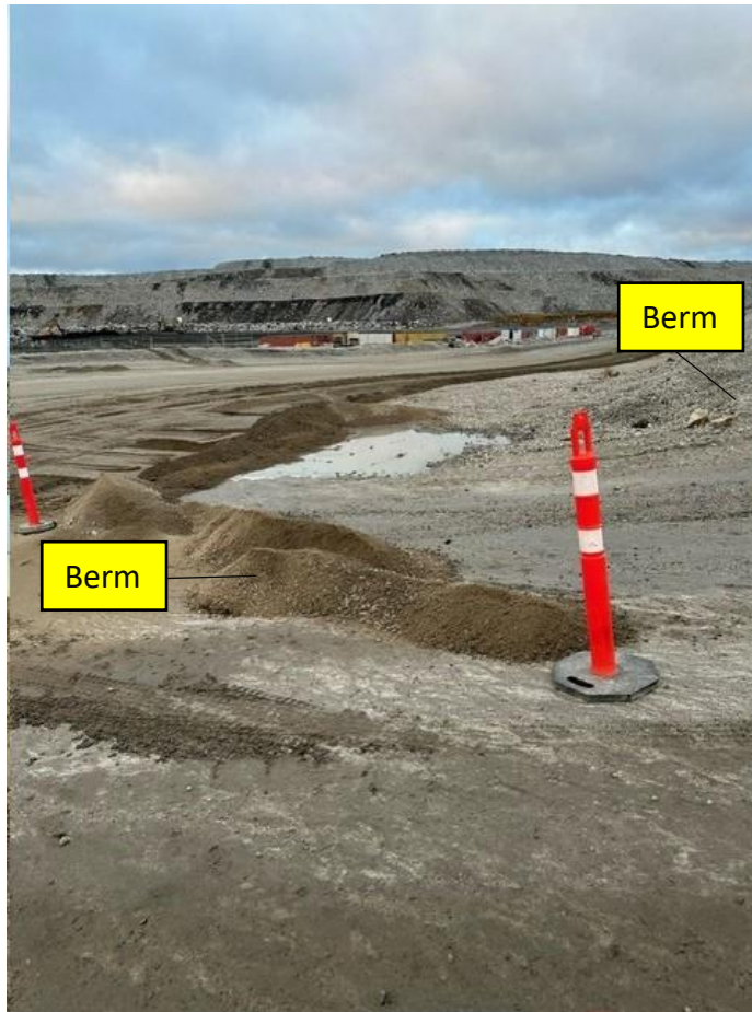
Photo 3. View of berms made directly adjacent to the fuel station to contain the diesel fuel spill. Photo facing north.
