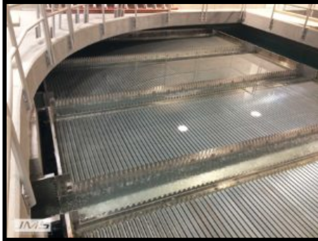
Figure 4. WTP plate settlers (Jim Myers & Sons, Inc., 2019)
