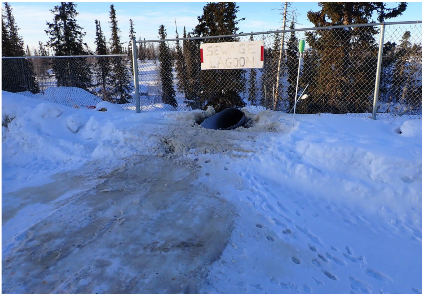
Figure 2. Sewage Lagoon Off-load Location
