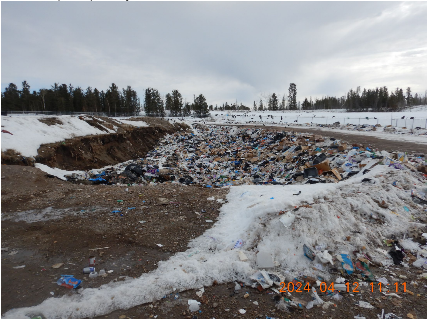
Photo 6: Trench pit for disposal of regular household waste.
