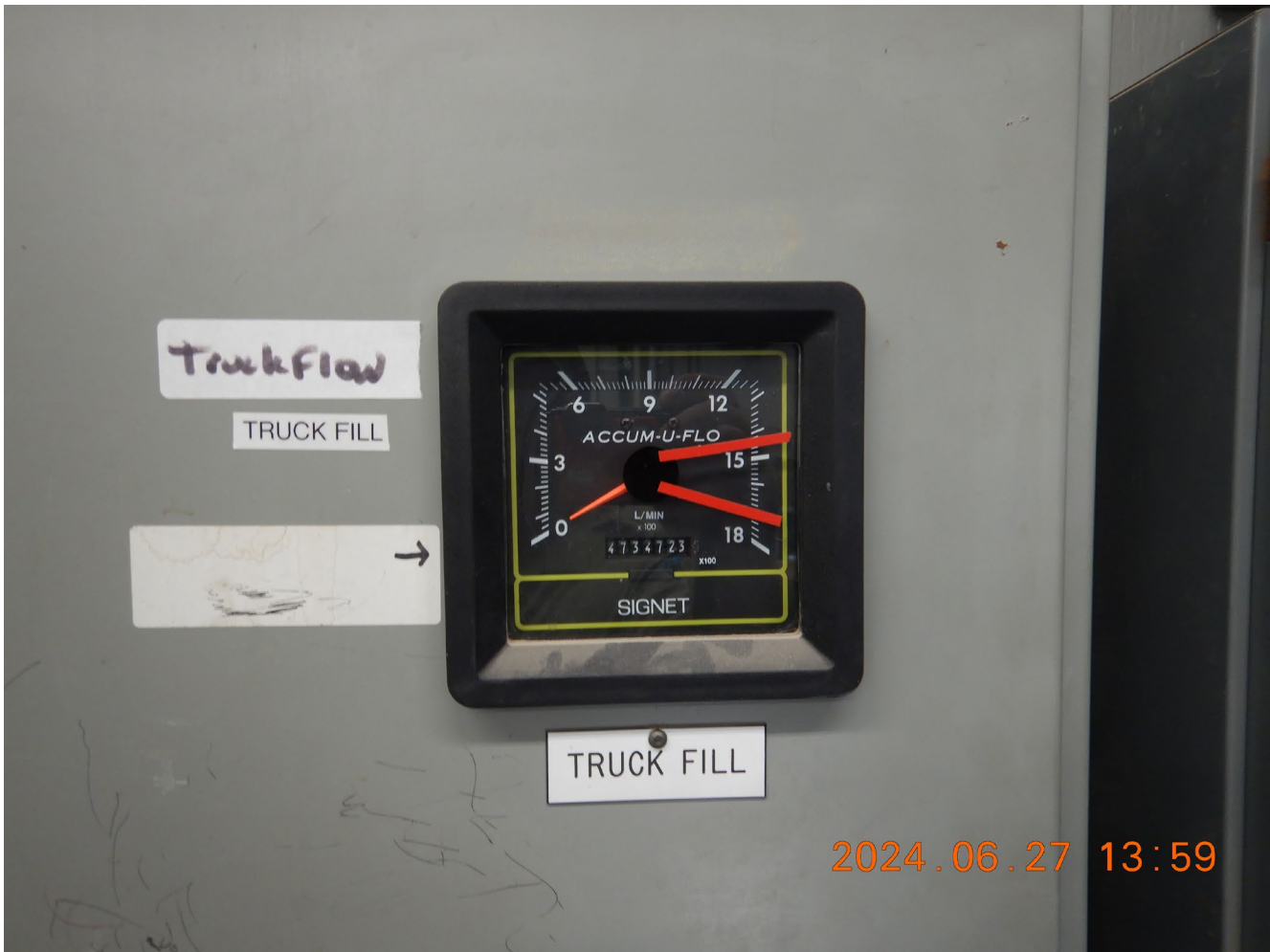
Photo 2: Meter for trucked water.
