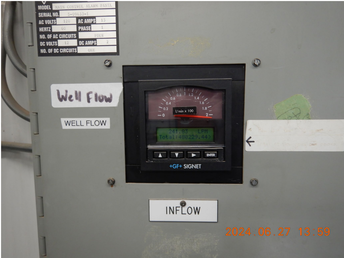
Photo 2: Meter for trucked water.
