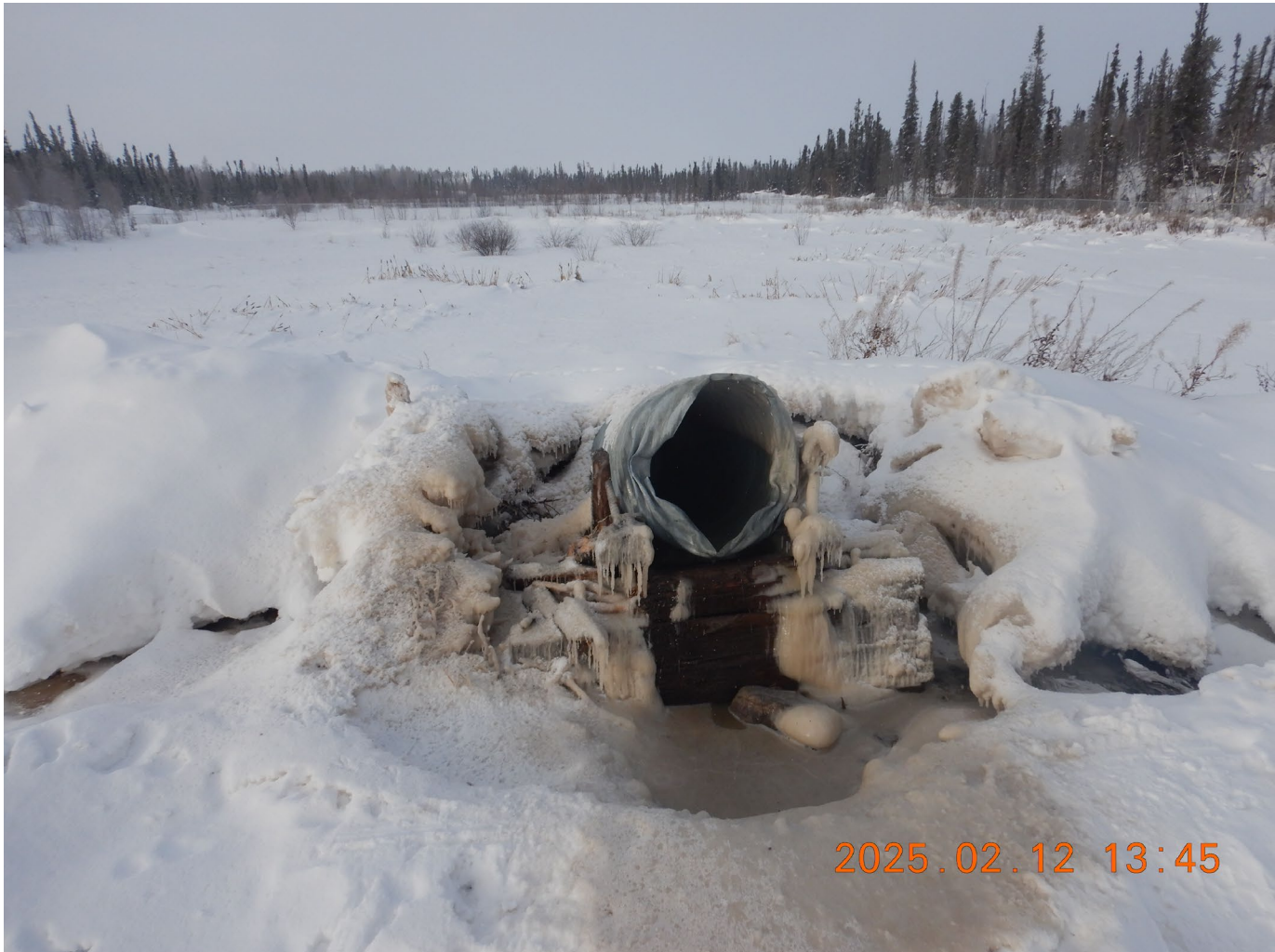
Photo 4: Lagoon. Better efforts to direct sewage to the primary cell must be made.
