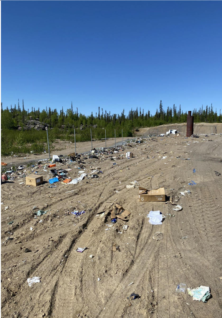
Figure 3 - Windblown waste and missing fencing
