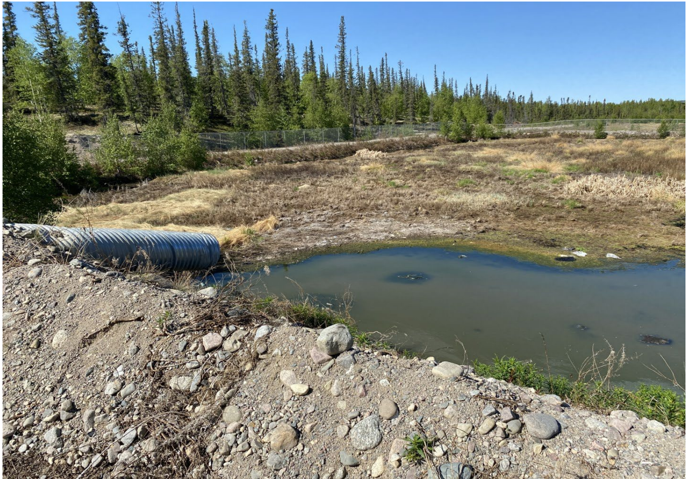
Figure 1 – Discharge location and infiltration berm
