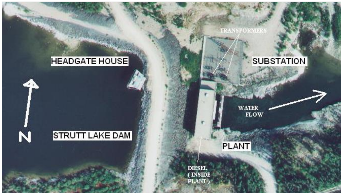
Figure 2-5: Snare Forks Hydroelectric Facility
