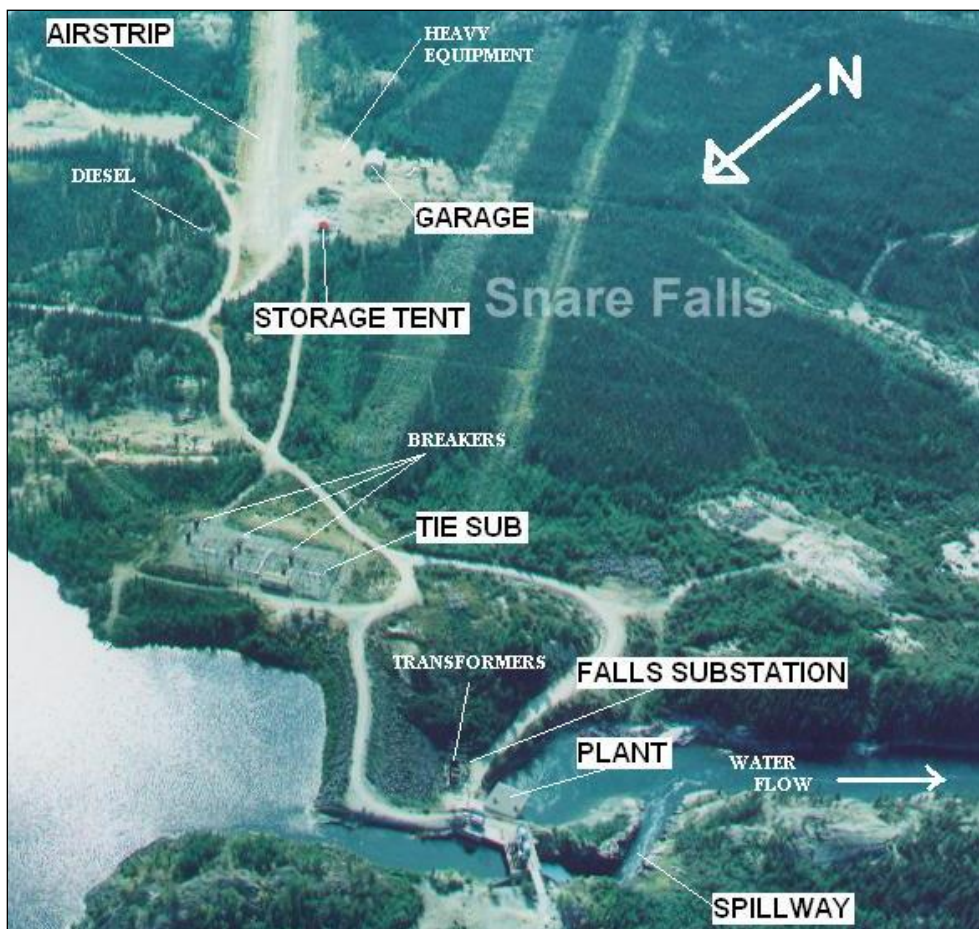
Figure 2-3: Snare Falls Hydroelectric Facility
