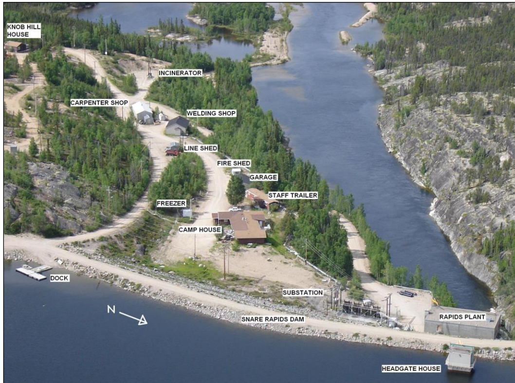
Figure 2-2: Snare Rapids Hydroelectric Facility
