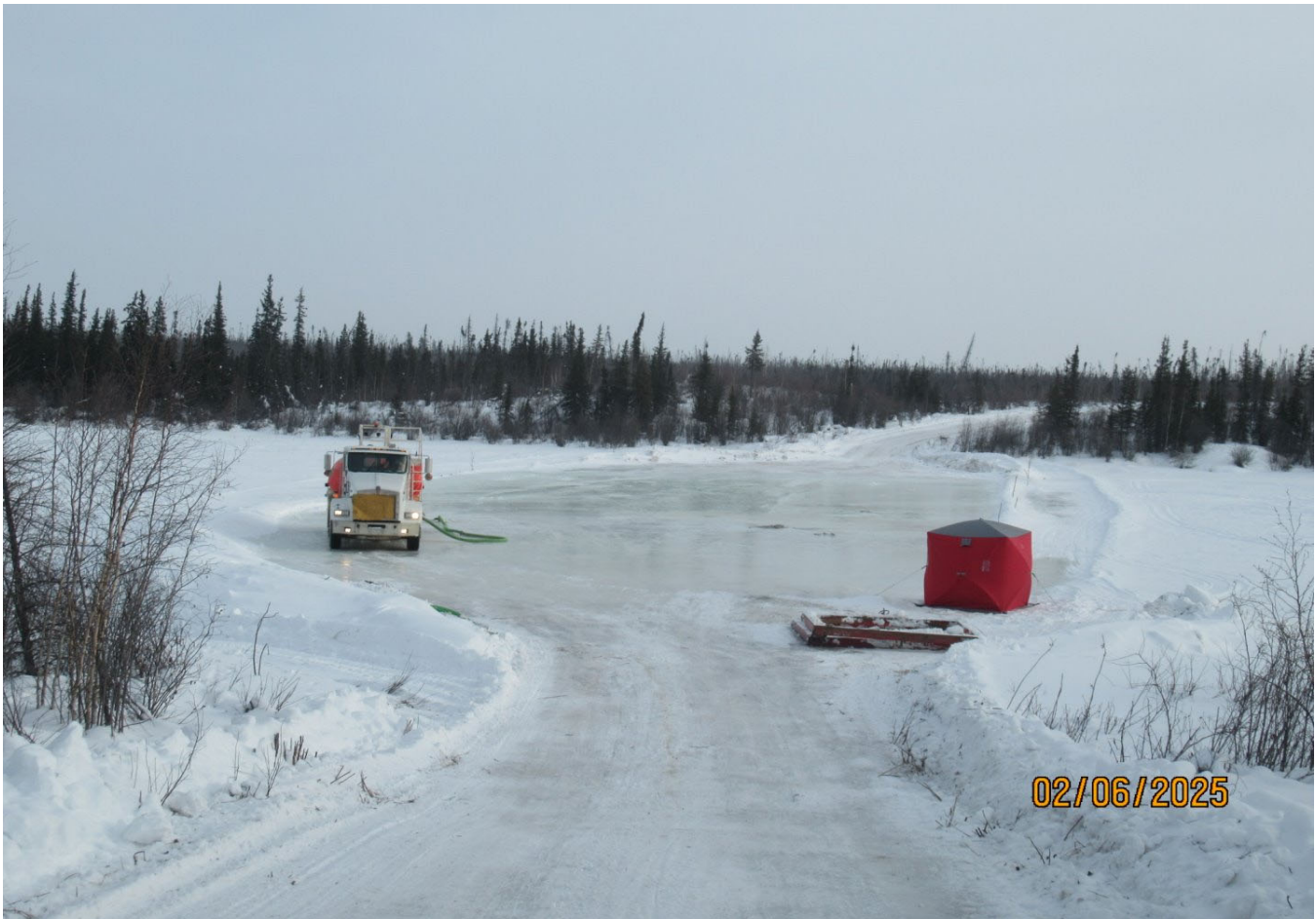
Figure 6 Example of a portage with initial icing completed. Final grooming must be completed to ensure icing from shoulder-to-shoulder of the right-of-way.
