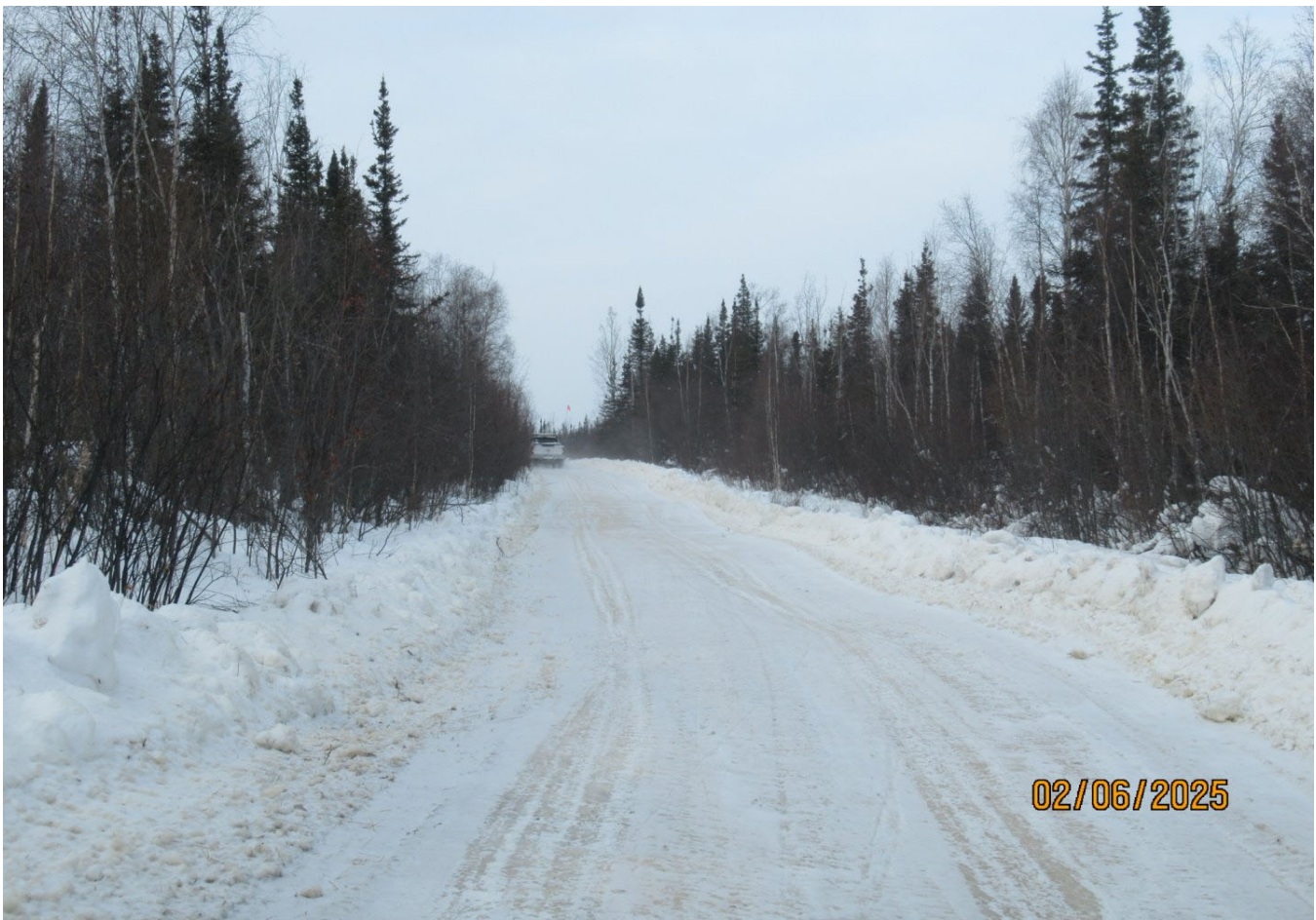
Figure 6 Example of a portage with initial icing completed. Final grooming must be completed to ensure icing from shoulder-to-shoulder of the right-of-way.
