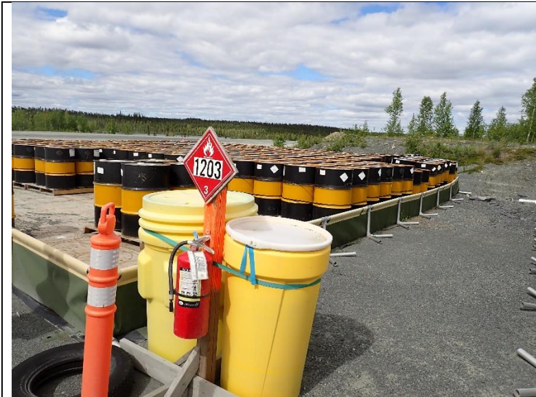
Photo #8: Close up of fuel storage located near the airstrip and spill kits located nearby.
