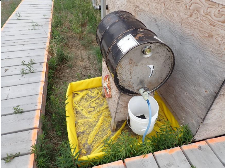
Photo #2: Fuel drum appropriately placed in secondary containment.
