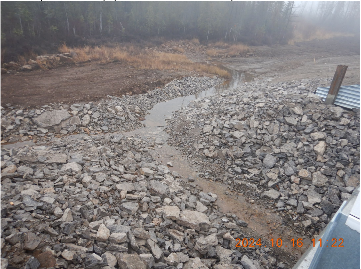
Photo 2: Completed installation. Rip rap has been installed in the streambed to prevent erosion.
