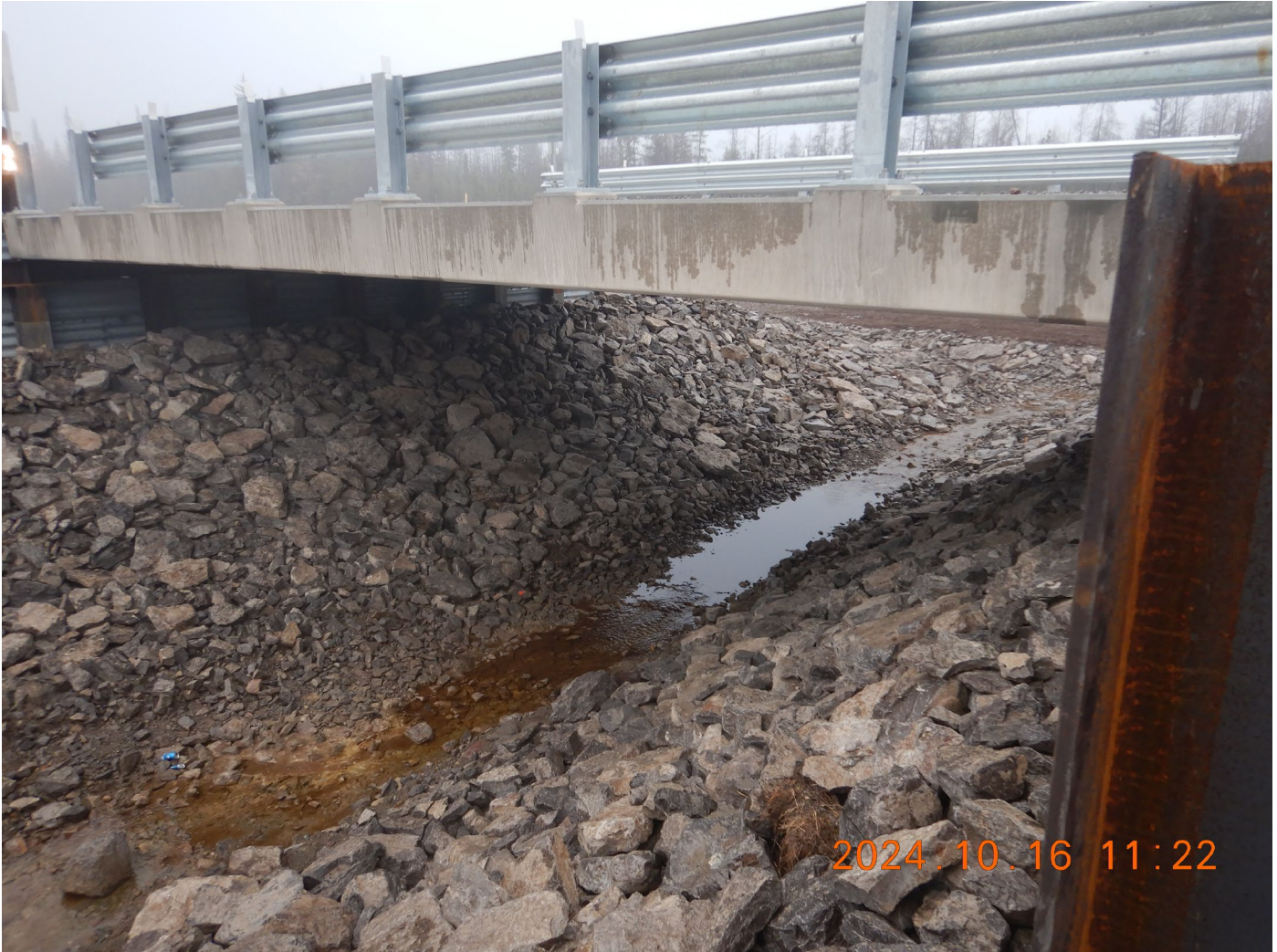
Photo 2: Completed installation. Rip rap has been installed in the streambed to prevent erosion.
