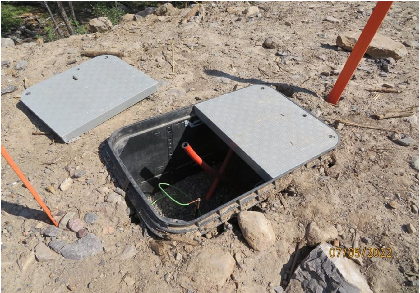
Figure 2 The Km #89 pull box, showing very minimal disturbance.
