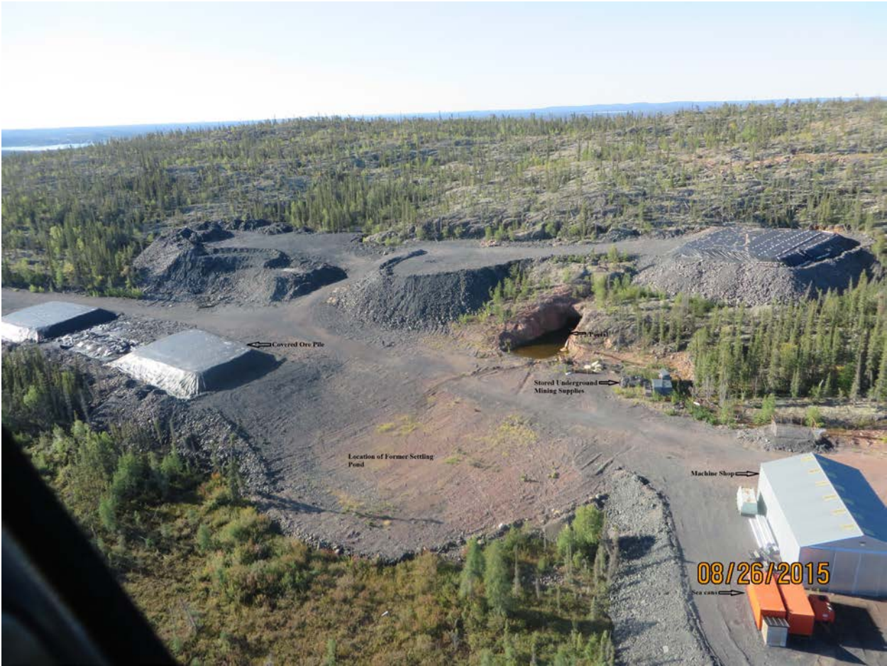
Photo 2. Underground Exploration Area (close up)
