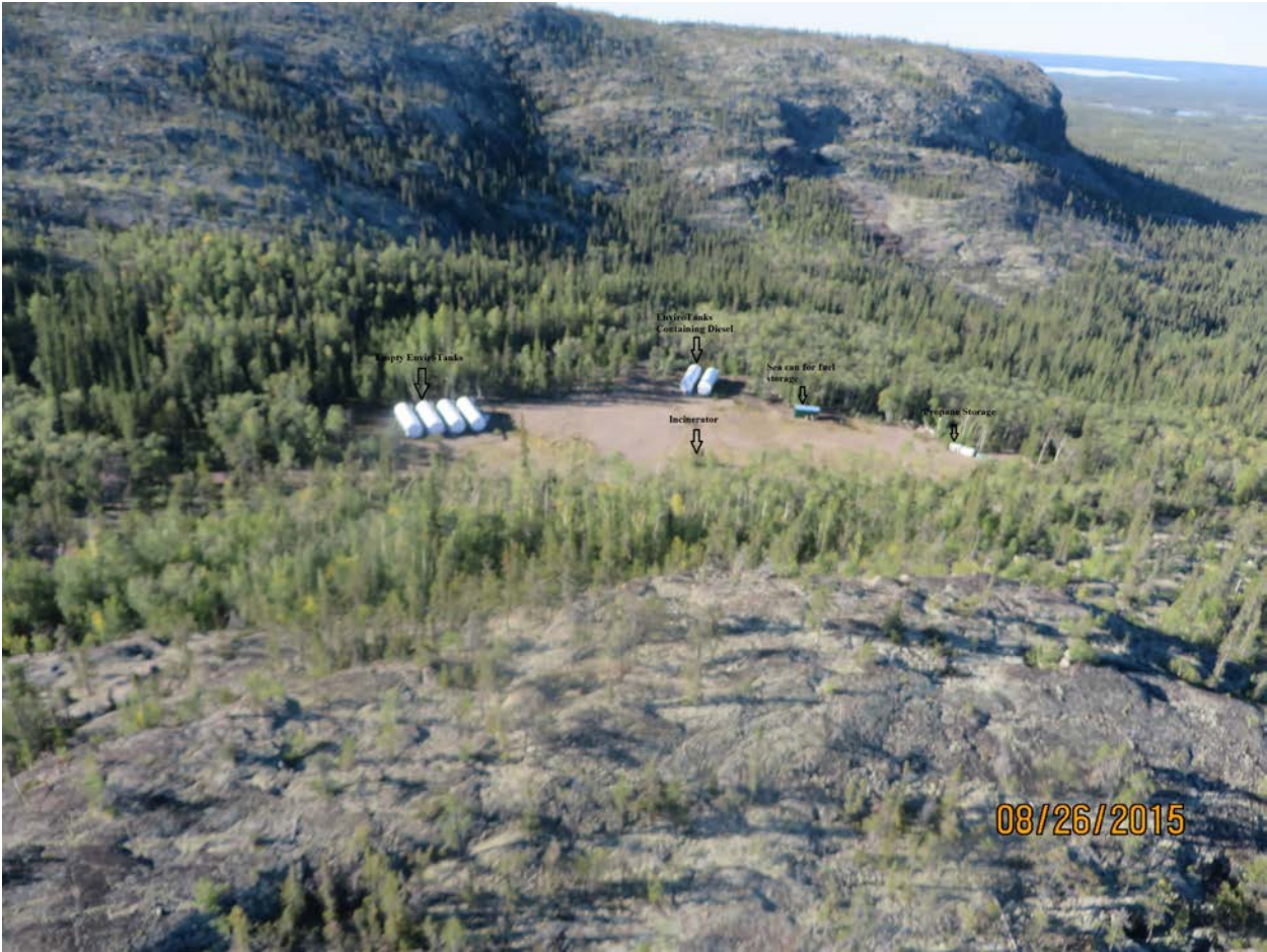
Photo 3. Fuel Storage Area
