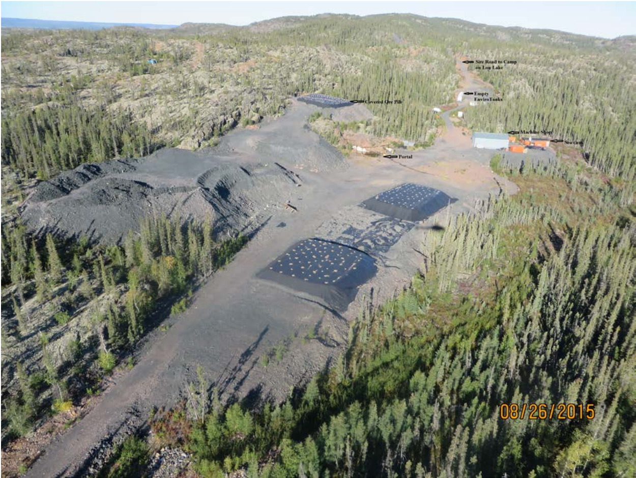
Photo 1. Underground Exploration Area.
