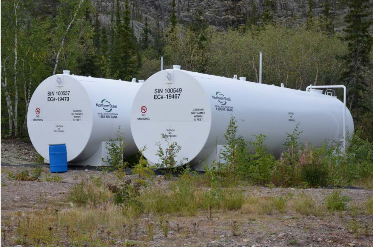
Photo 6: EnviroTanks with diesel (SIN 100557&SIN 100549)
