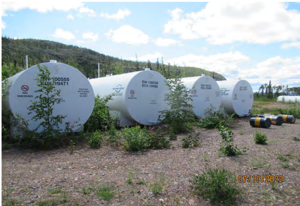
Photo 6 Four EnviroTanks with fuel farm. Note: fuel barrels on the ground have since been removed
