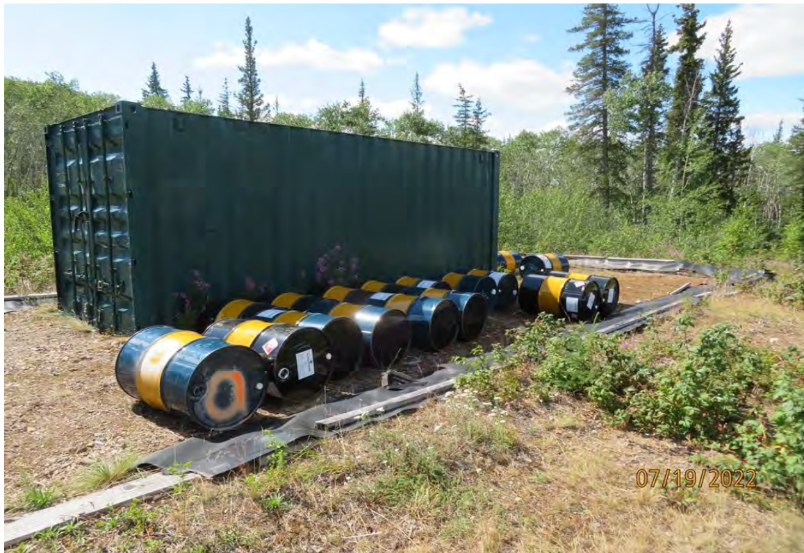
Photo 6 Four EnviroTanks with fuel farm. Note: fuel barrels on the ground have since been removed
