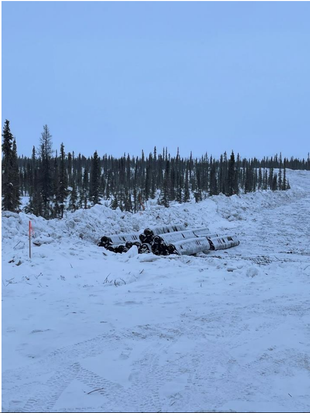
Photo Description: Geotextile on Site
