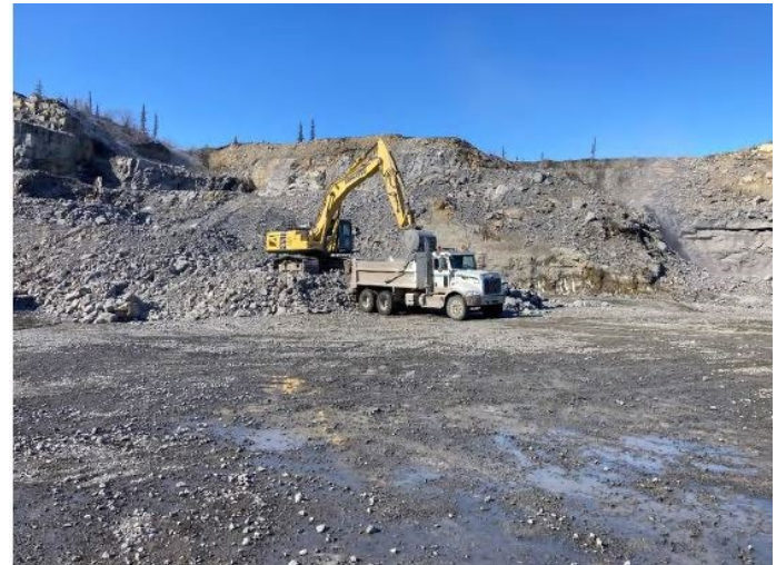
Loading Material at Quarry
