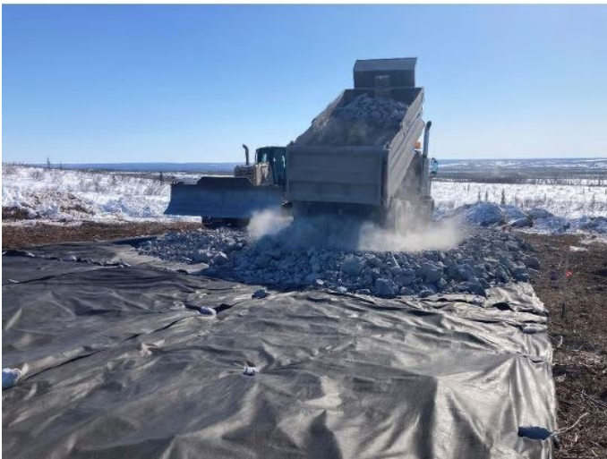
Placing Blasted Material
