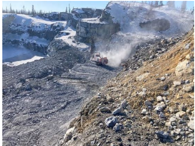
Drilling Blast Area #4
