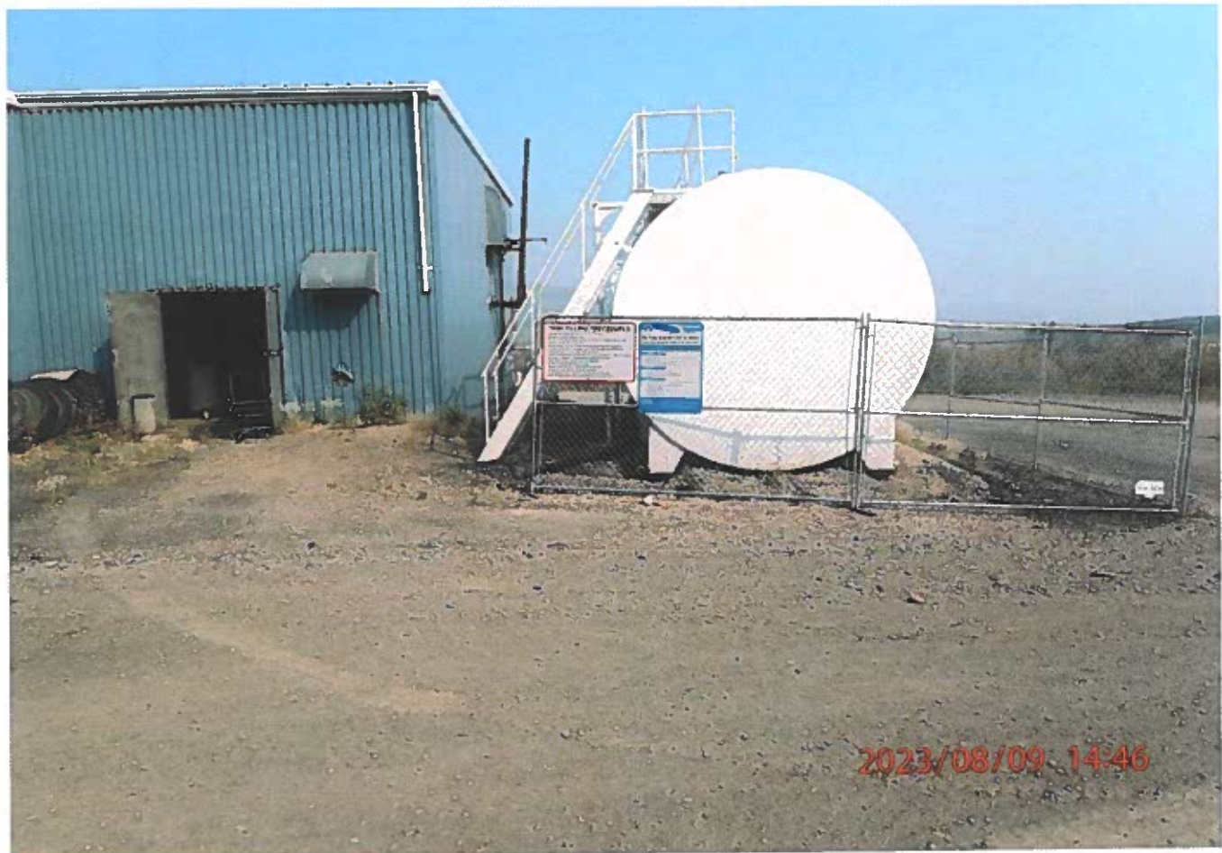
The back side of the fuel storage tank.
