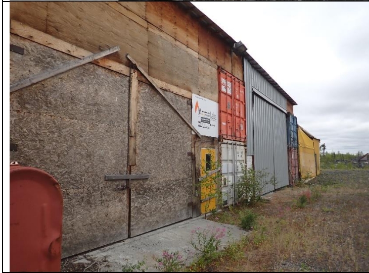
Photo #8: Portal shop continues to be secure
