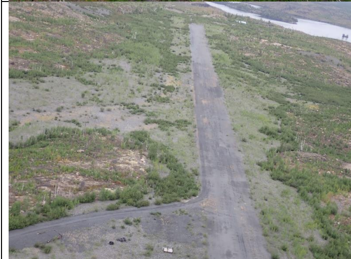
Photo #3: Overview of the airstrip
