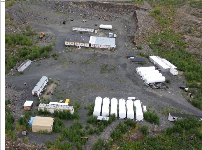
Photo #2: Overview of the camp and fuel storage
