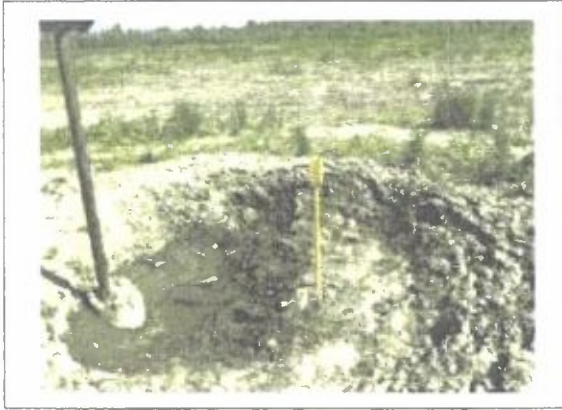
Well centre facing east.
