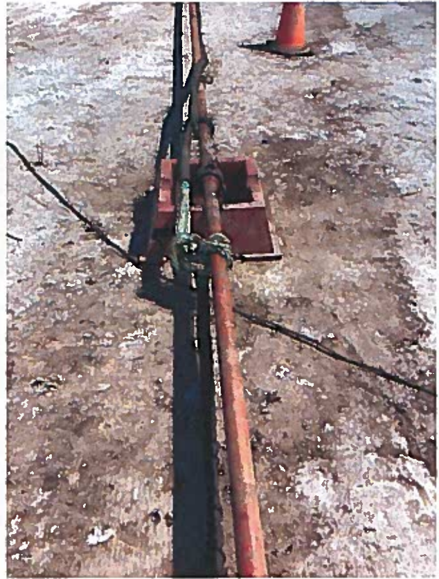
Photo # 10: Flow line and choke lines secured.
