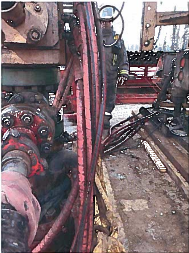
Photo # 3: Fire rated kelly hoses within 7m from the BOP.
