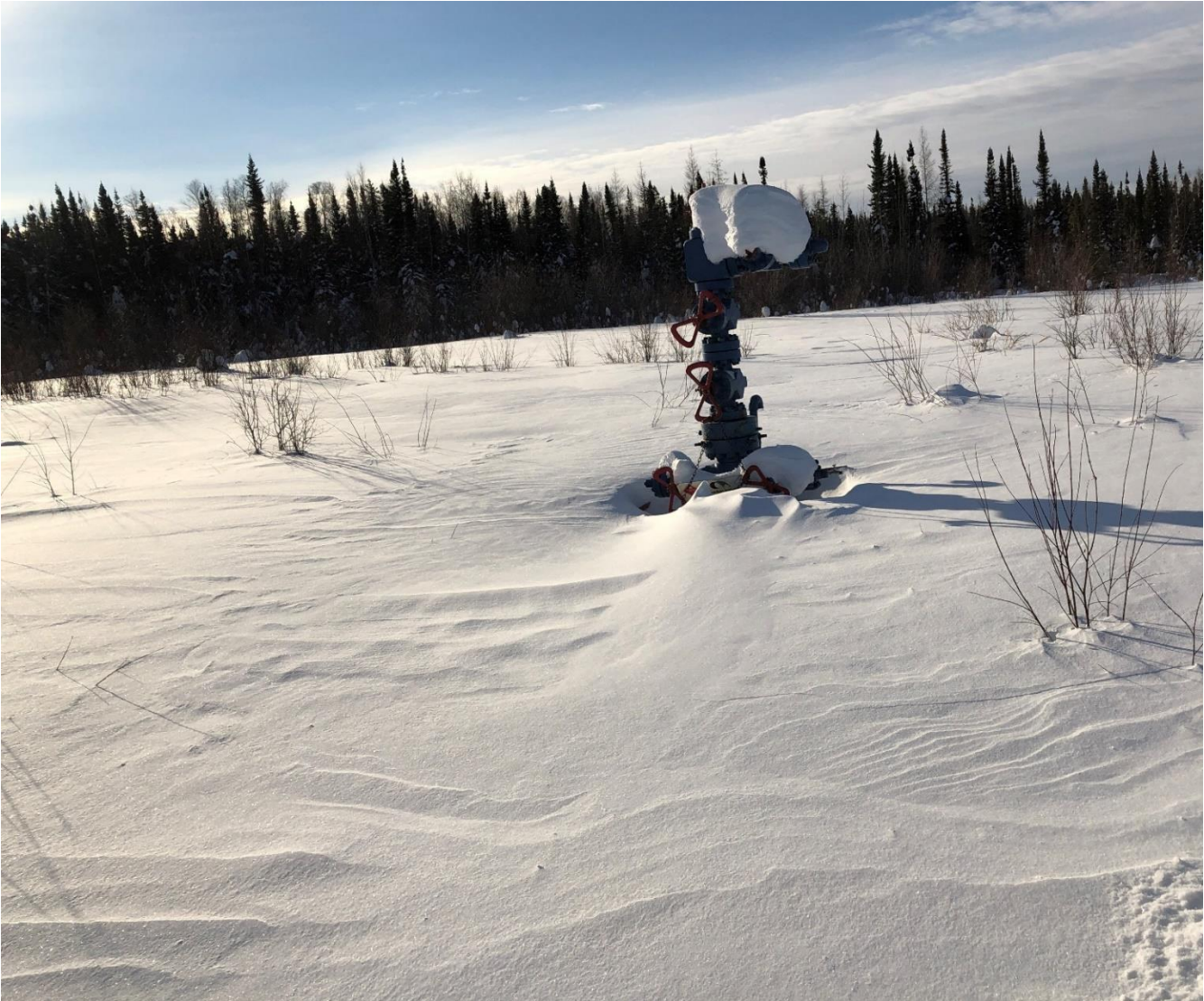
Photo #2: Well head Netla C-07 – No wind indicator – Brush encroachment on wellhead
