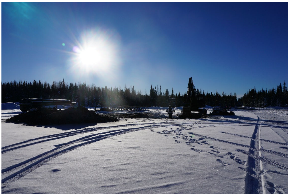
PHOTO #2: Overview of the operations on site.
