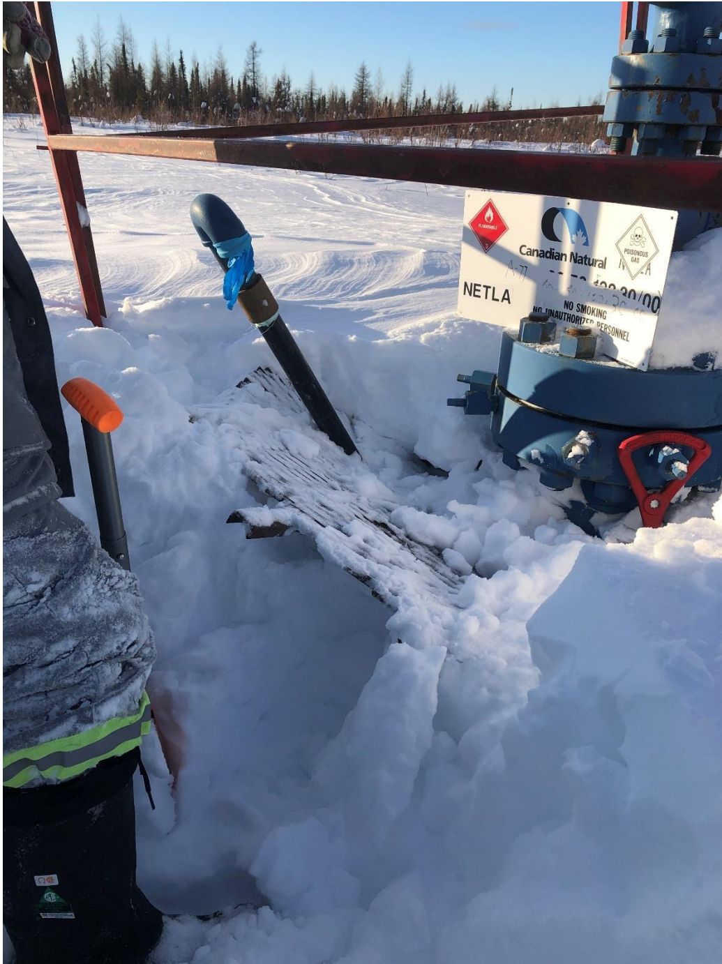
Photo #3: Emile Lake A-77 - Well head identification sign – Surface Casing Valve not accessible
