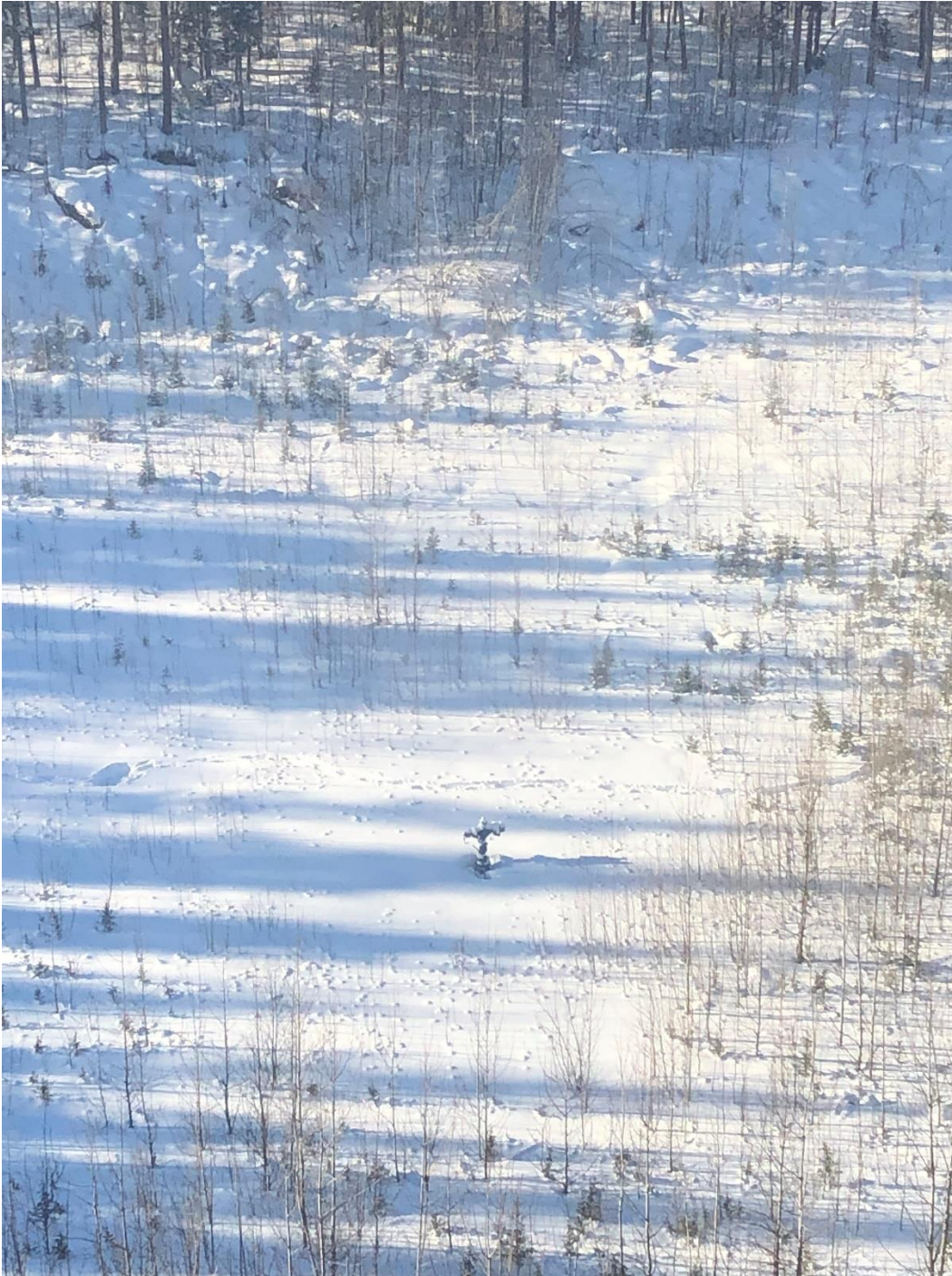
Photo #2: Aerial view of Liard P-16 Well Head – Vegetation Encroachment
