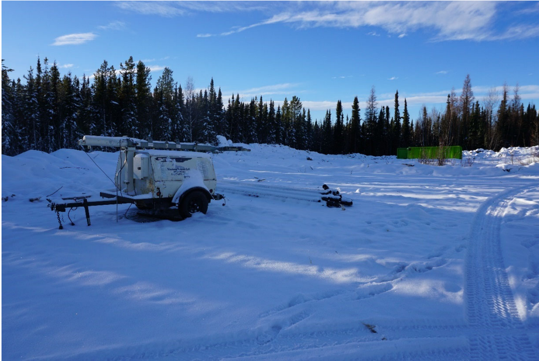
PHOTO #3: Equipment staged on site that must be removed after cut and cap operations are complete.
