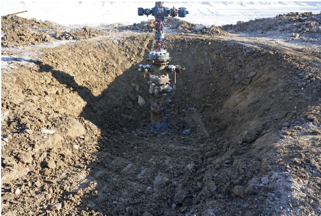
PHOTO #2: Material around the well head has been removed approximately 2 meters below ground surface.
