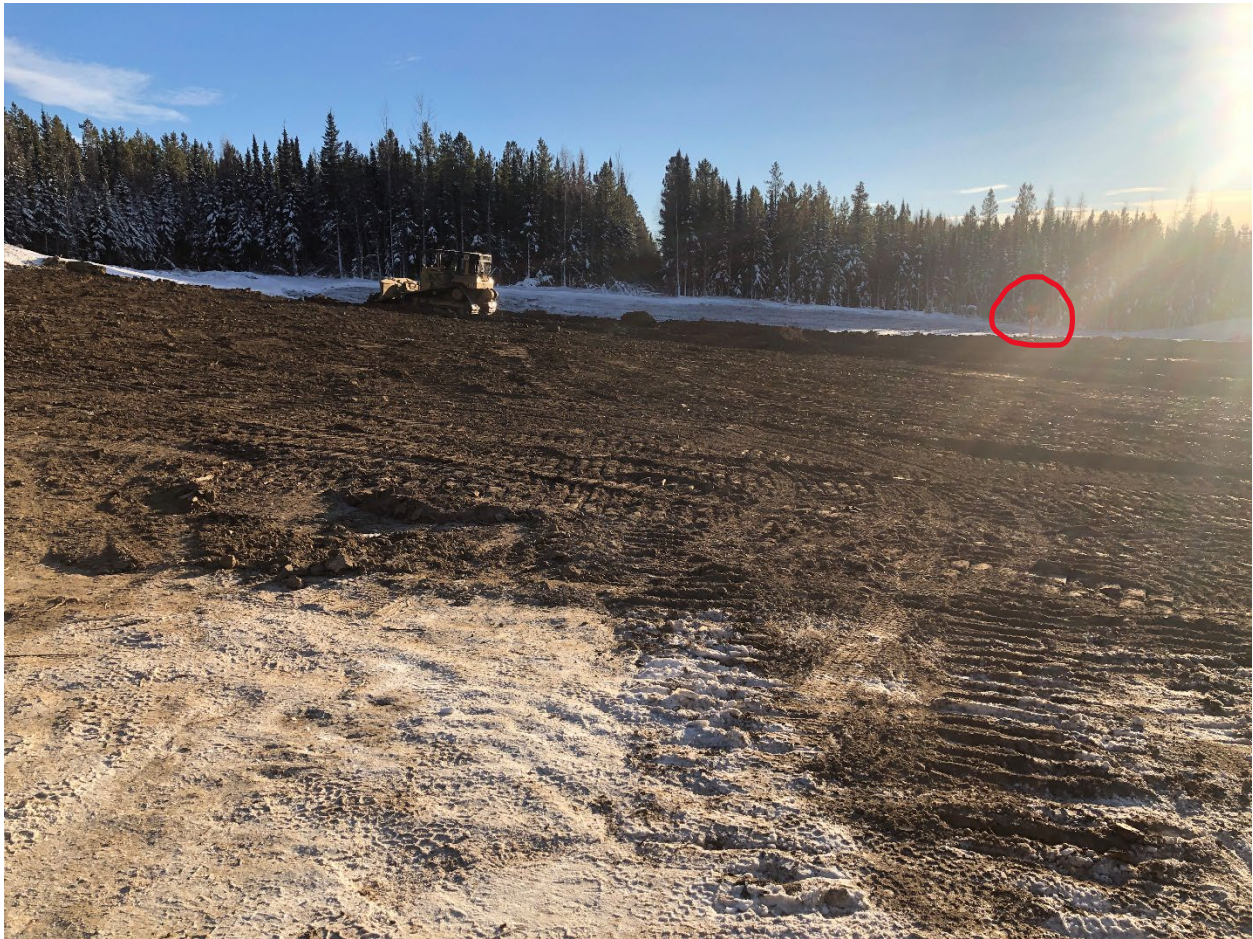
PHOTO #1: Site being recontoured. Well abandonment sign in place
