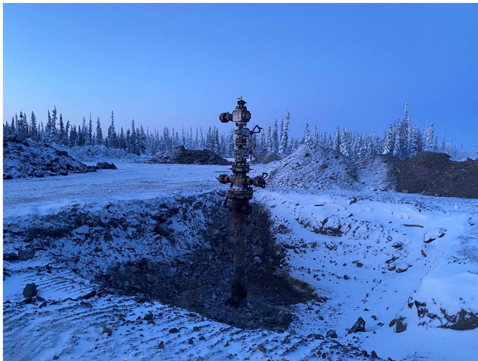
Photo 2: Nogha C-49 (WID1934) wellhead prepared for surface abandonment
