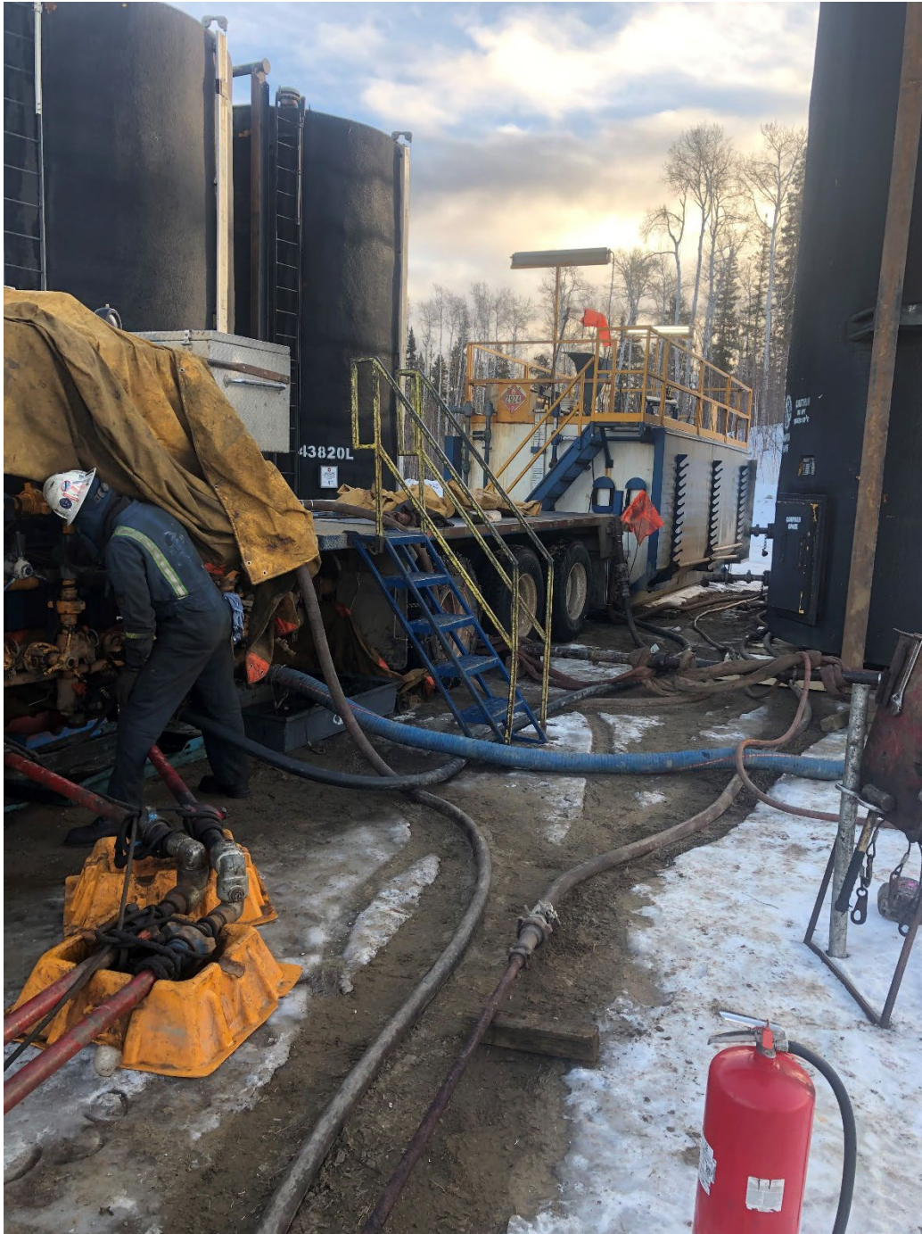
Photo #14: Rig pump to rig tank >7m.
