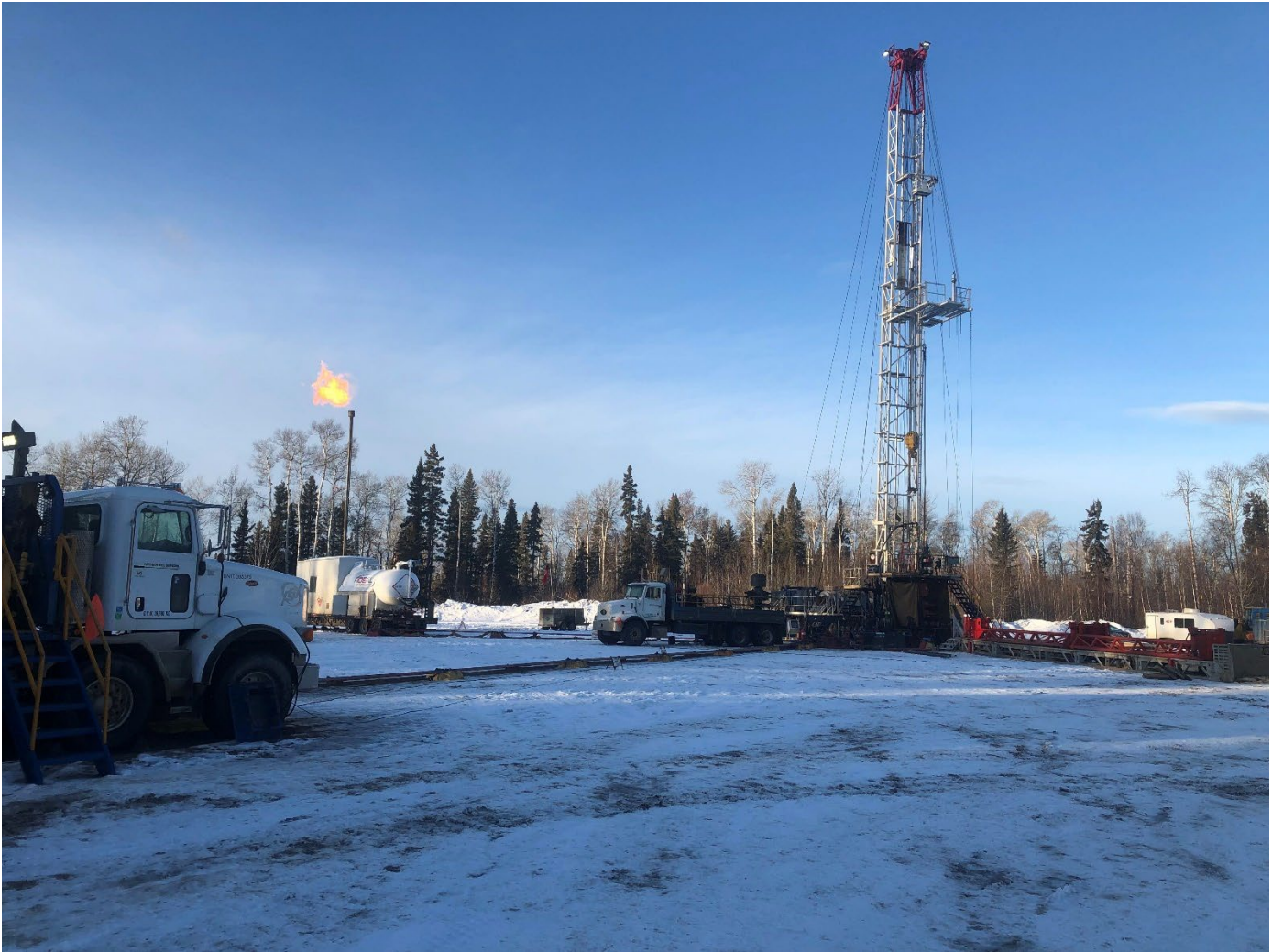
Photo #1: Mount Coty 2K-02 (WID 1993) well abandonment operations surface overview.
