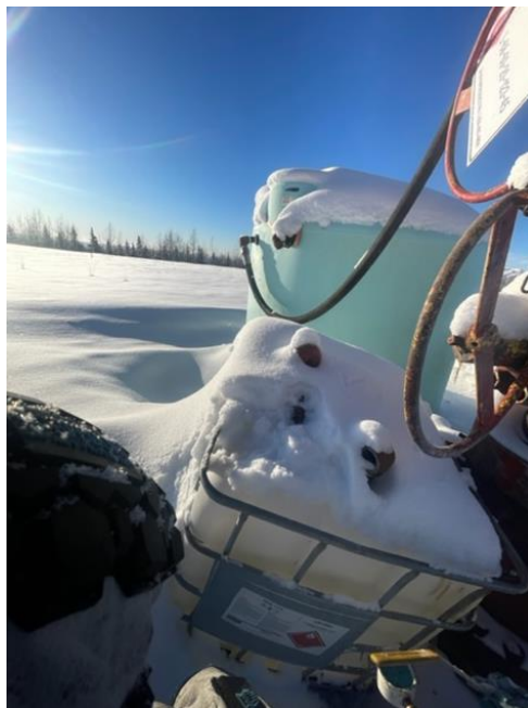
Figure 8 - PPR L-68 Wellhead (South)
