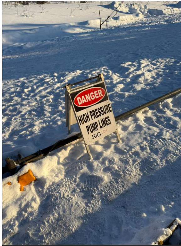
Photo 25: High pressure pump line signage
