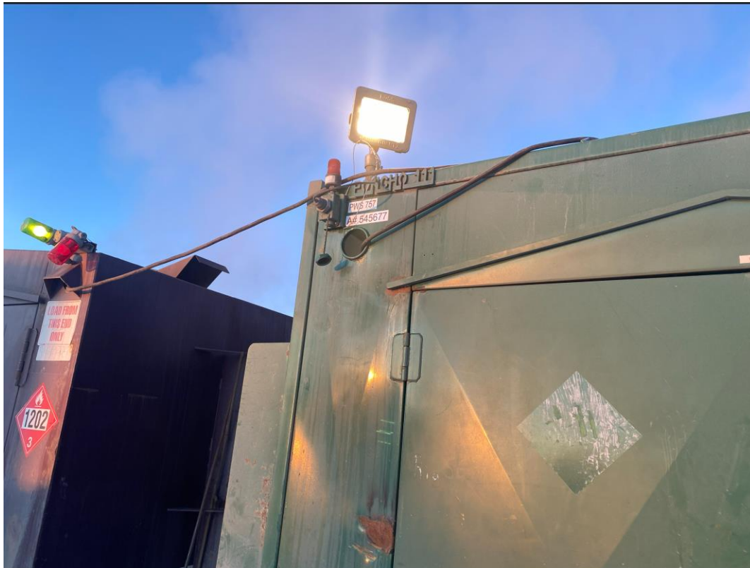
Photo 8: Boiler PWS 757 (out of service)
