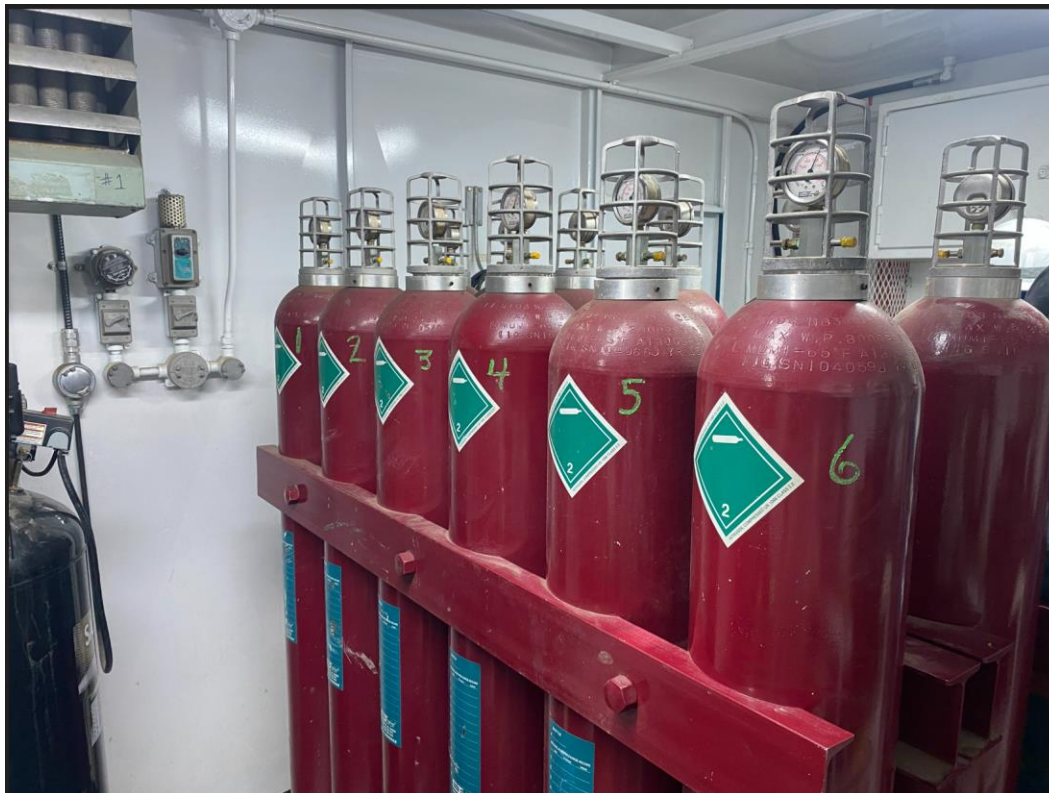
Photo 4: Accumulator bladdered nitrogen bottles
