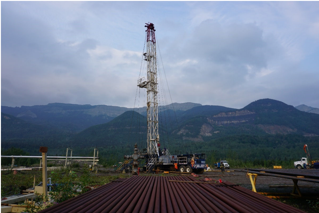
Photo #10: Rig matting placed below the rig during active operations.
