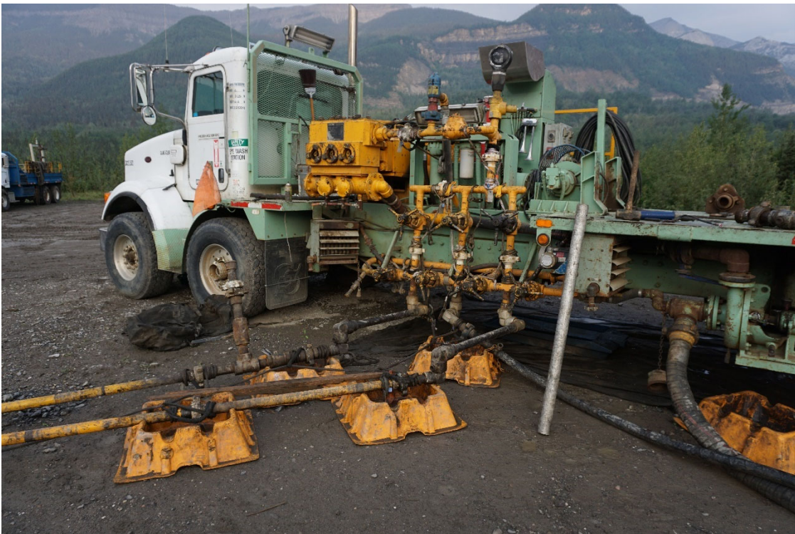
Photo #5: Pump lines secured, flow turns are in the correct position.
