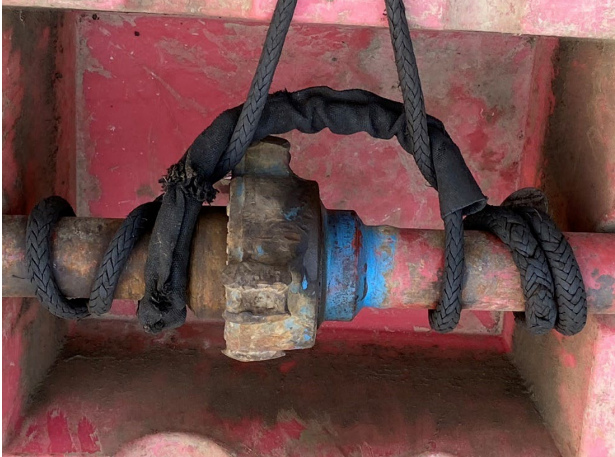
Photo #6: Flow lines secured
