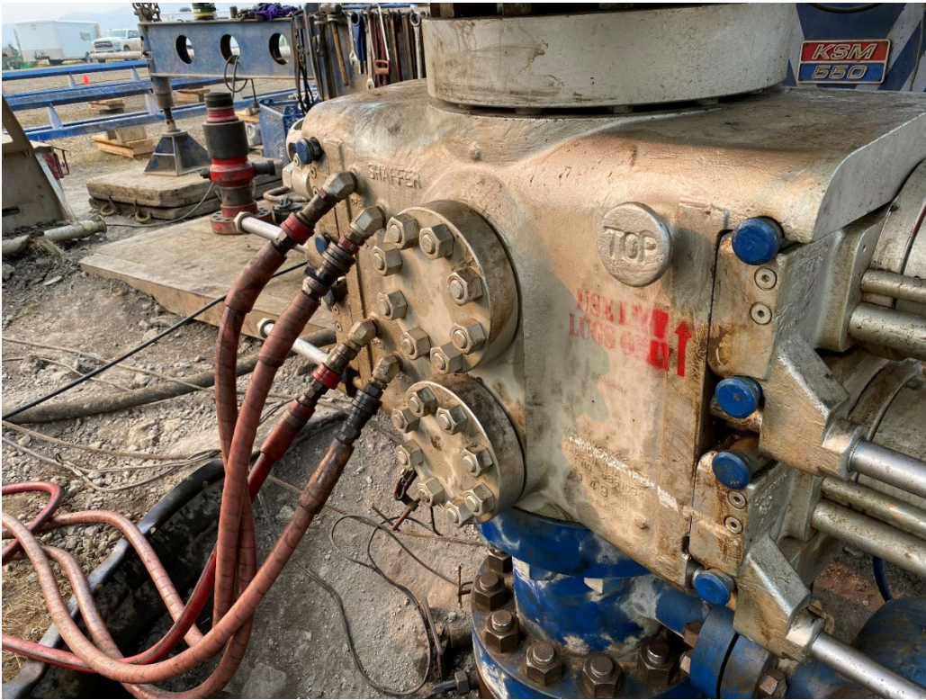
Photo #3: Double Gate in use on site
