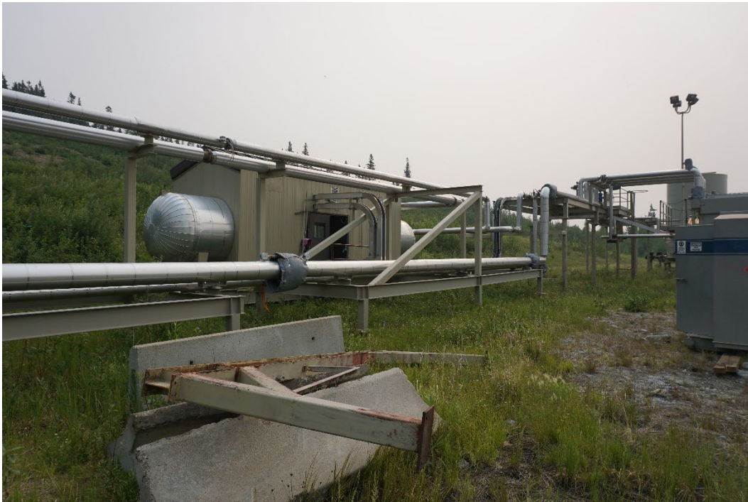
Photo #11: Installations on site
