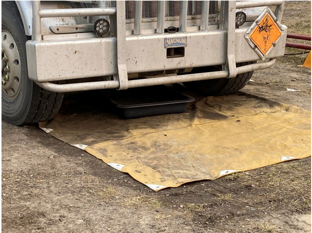
Photo #10: Drip trays in place under equipment
