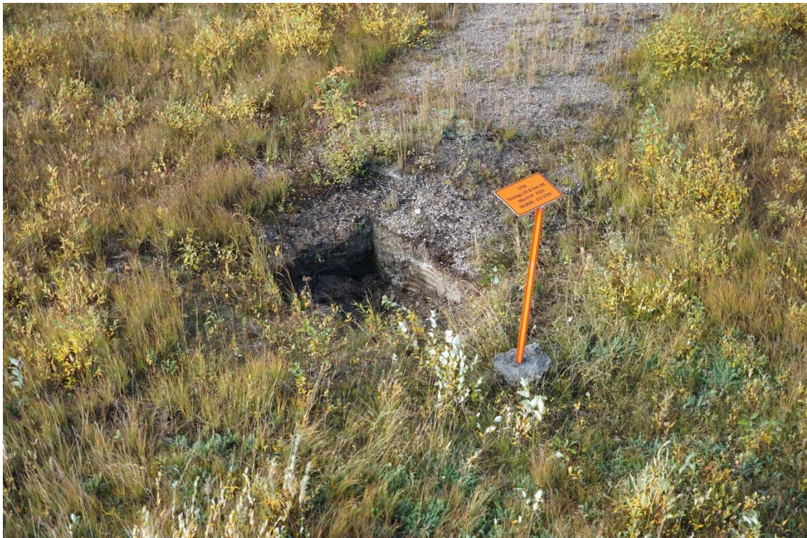
Photo #2 Close up view of the well center which has not been backfilled and mounded to prevent the ponding of water. The well sign is also bent over and may fall off in the near future.
