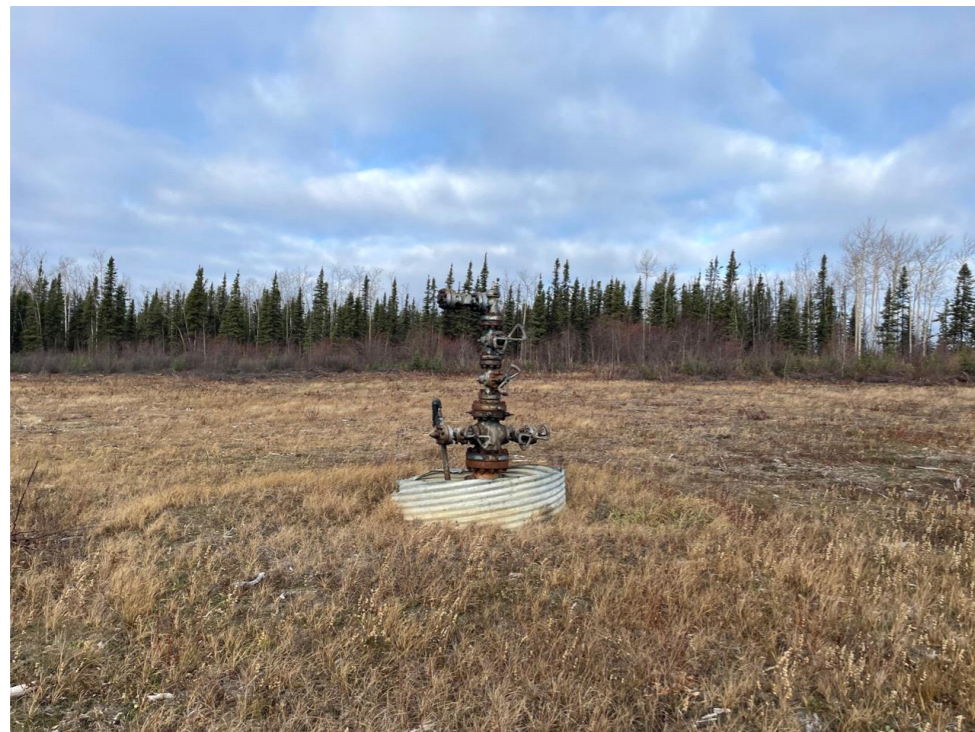
Looking South at well centre
