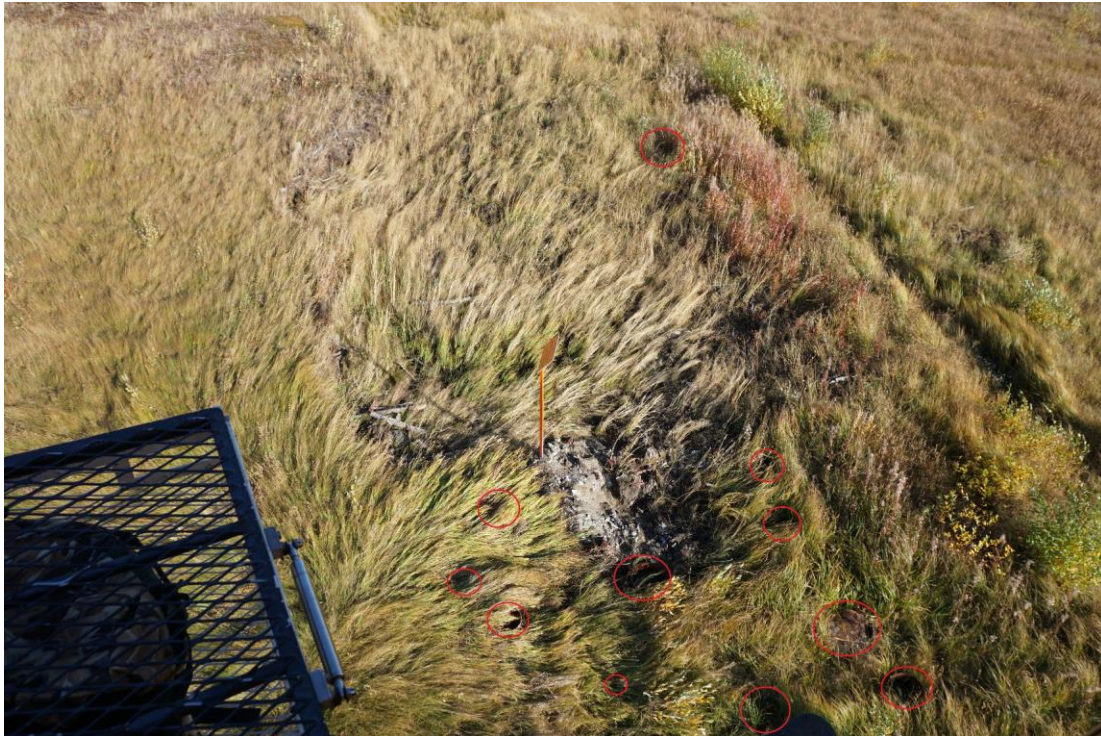
Photo #1: Cameron 2H-03 (WID2073) – 11 identified unsecured pilings circled in red
