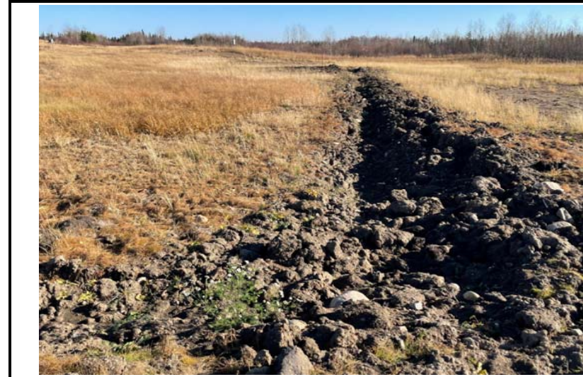
East towards well centre showing trench where flowline was (removed Feb 20, 2023)
