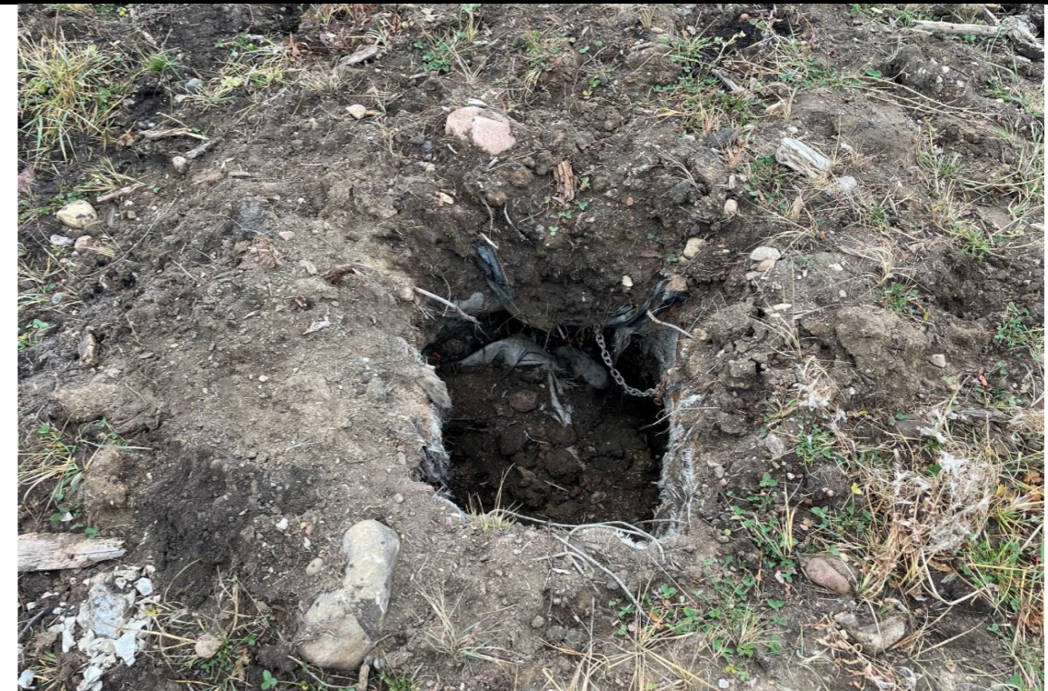
Subsidence at well centre from cut and cap. Removed as much loose debris as possible
