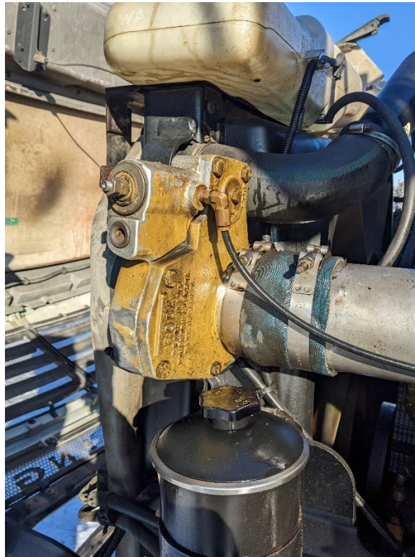
PHOTO #11: Air cut off device that is part of the engine kill assembly.
