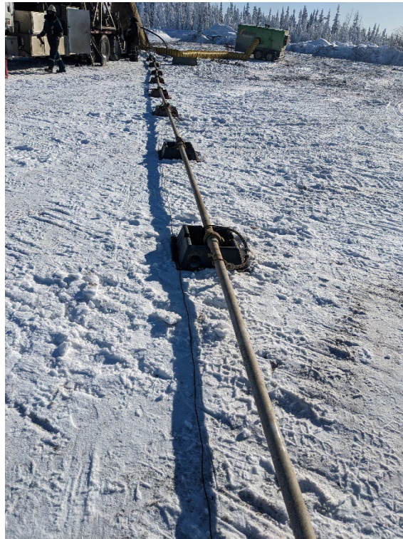
PHOTO #9: Pump line between well and rig tank.
