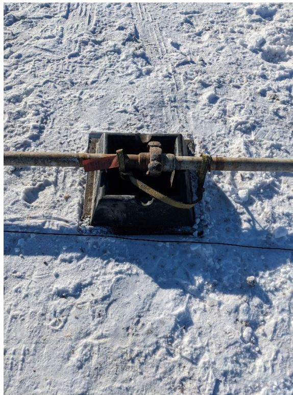
PHOTO #10: Pump line between well and rig tank secured between joints.
