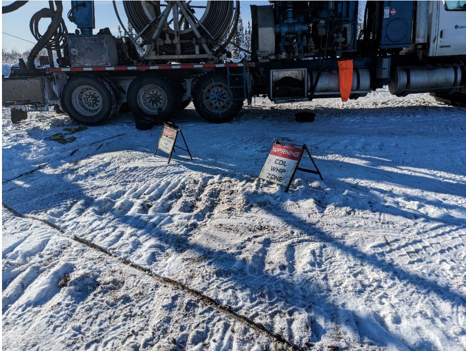
PHOTO #15: Hazard identification signs in place.
