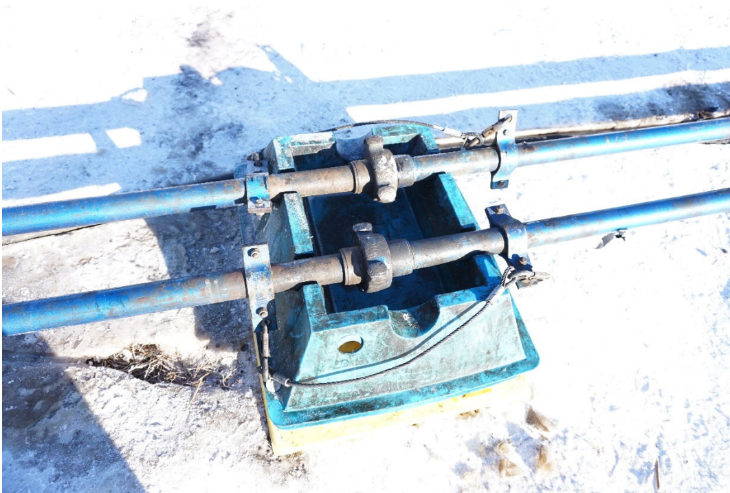
PHOTO #8: Lines from the Rig tank were secured.
