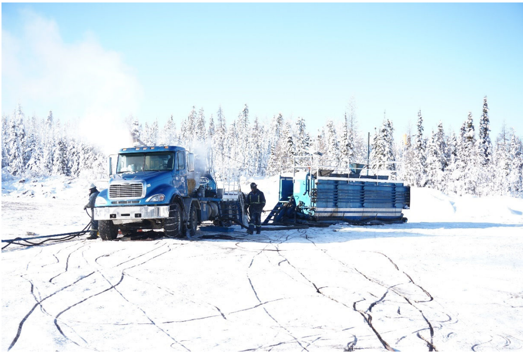
PHOTO #9: Although adequate room was available behind the rig tank to meet the minimum spacing requirements (50m), the rig tank was located 49.4m from the well center.
