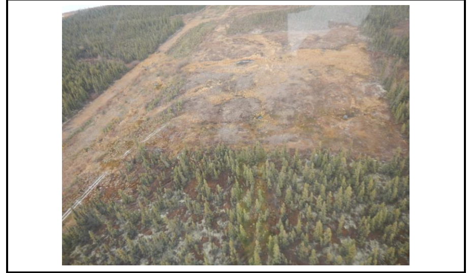
Looking northwest at lease from helicopter
