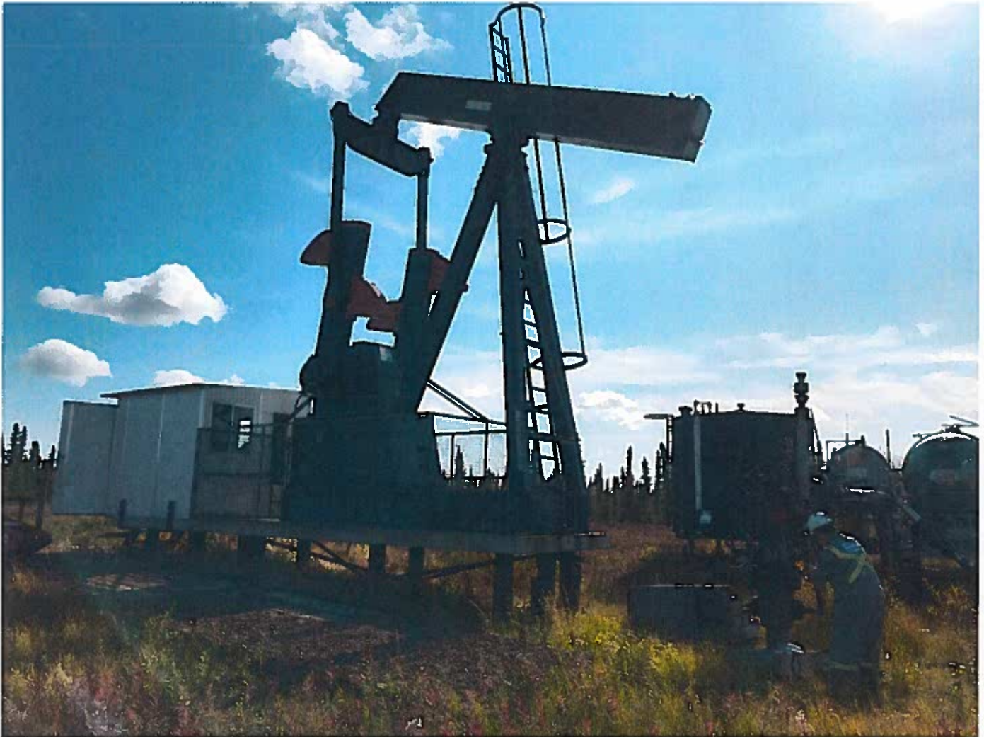
Photo # 1: Well Site - No wind indicator present on site. Wind indicator should be installed on well site.
