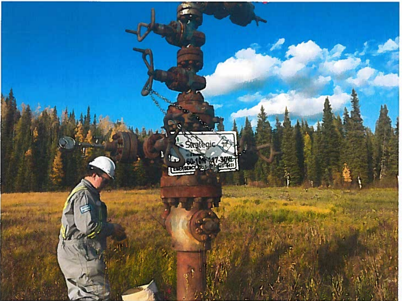
Photo # 2: Well site - Well head valves not secured. Key left in padlock. All well head valves must be secured to prevent unauthorized access.
