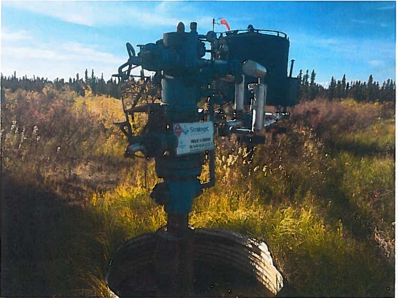
Photo # 1: Well Site
