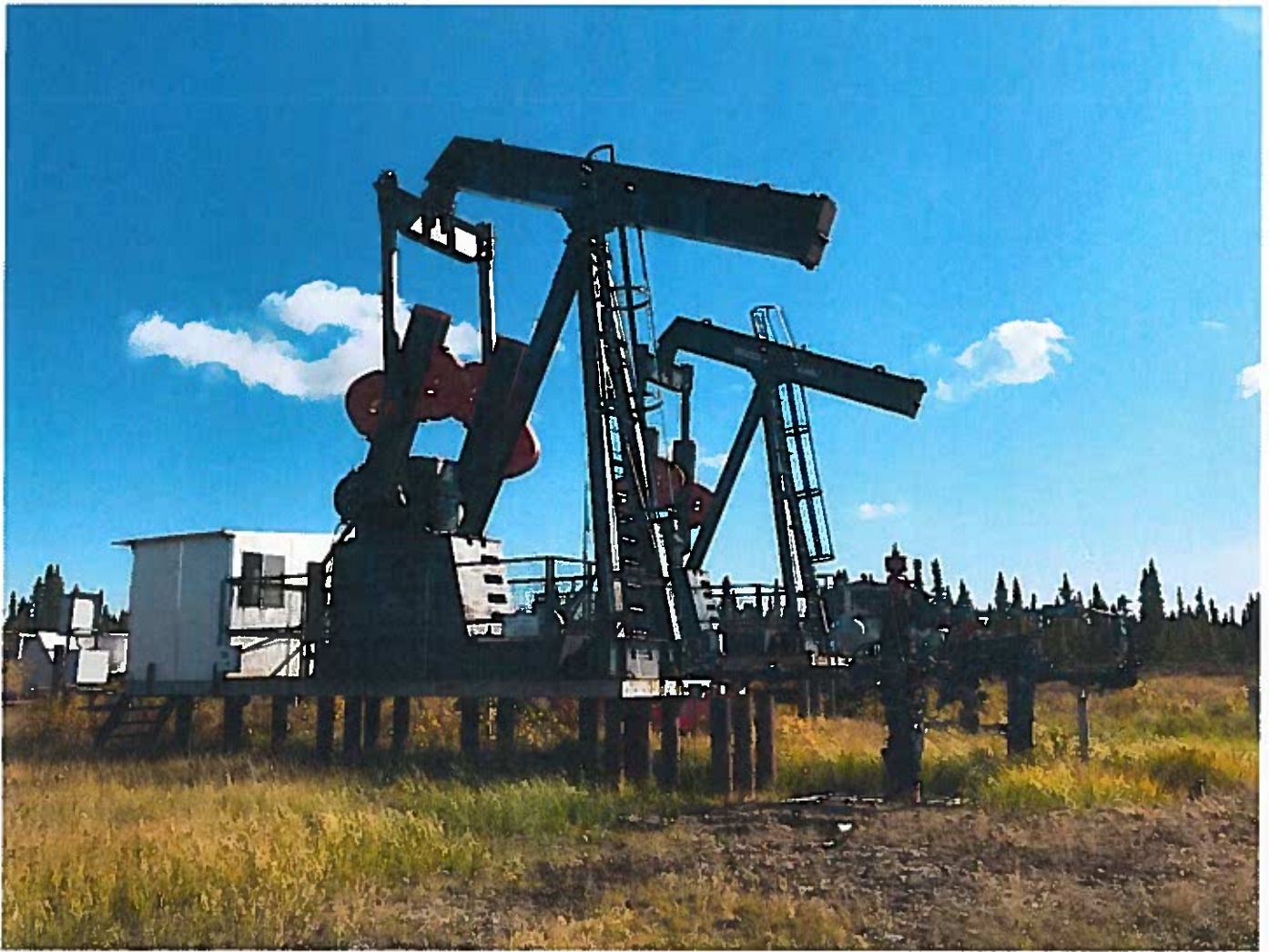
Photo # 1: Well Site
