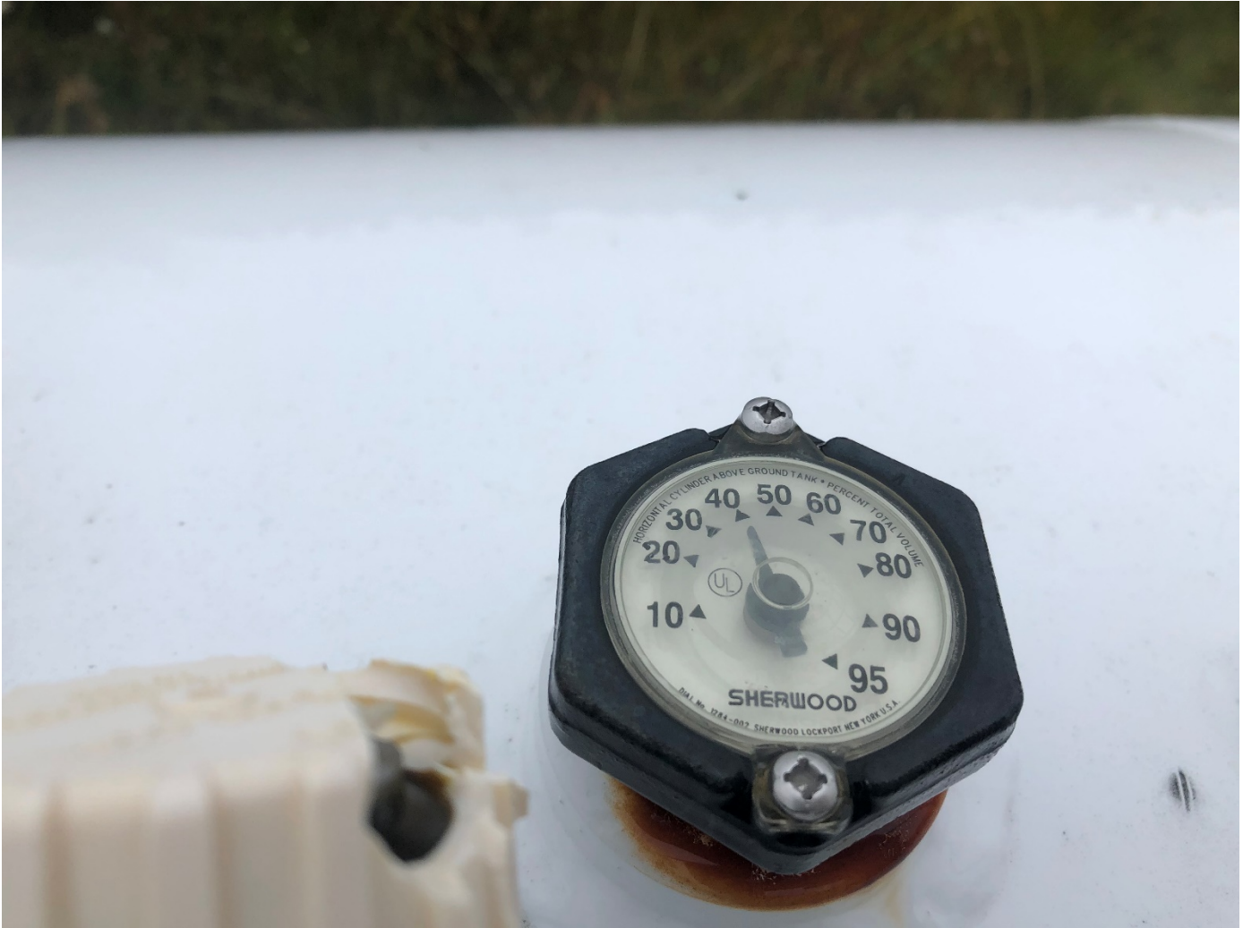
Photo #3: Propane vessel gauge reading approximately 40%
